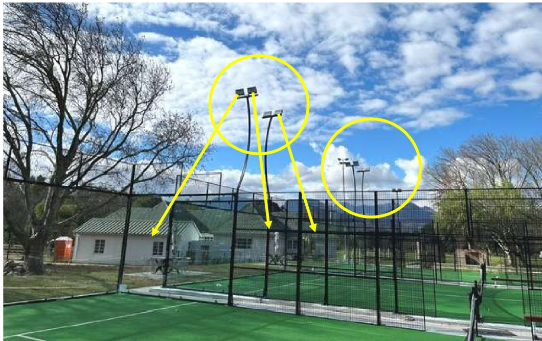
Padel courts with directional lighting
