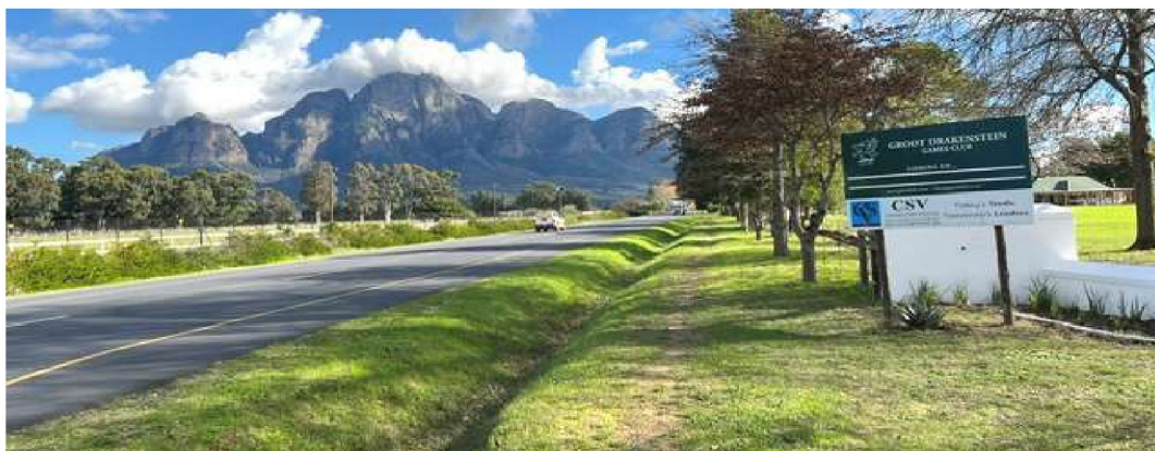
Western view onto the R45 from entrance
