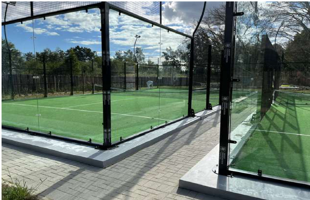
Padel courts on footprint of tennis courts
