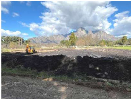
Detention pond under construction northeast of cricket oval
