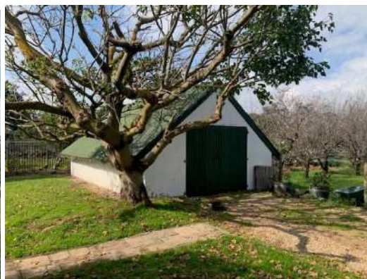
Shed near employee house
