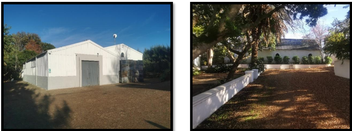
Figure 2: Photo of the existing wine cellar.
