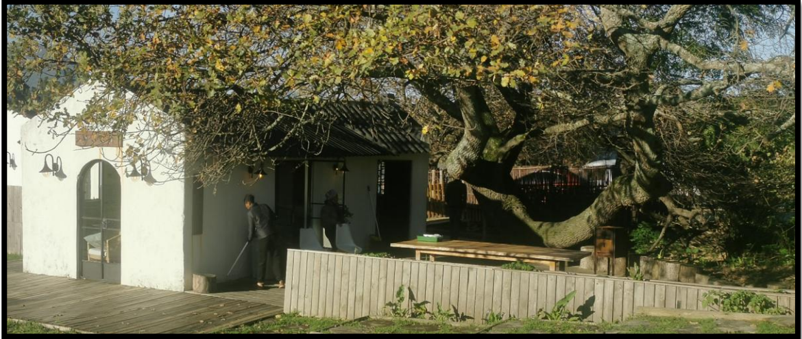
Figure 11: Photo of the service station.
