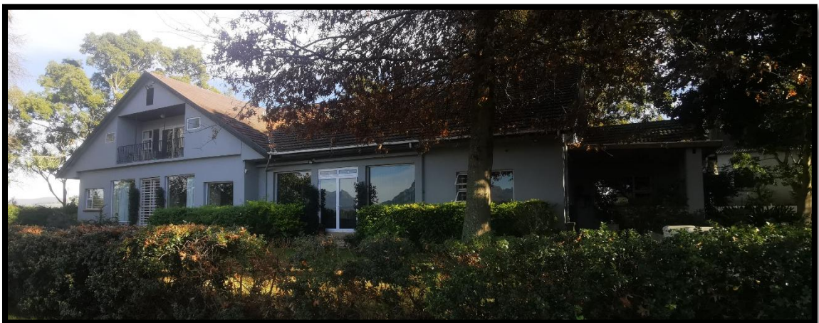
Figure 4: Photo of the existing Managers House.
