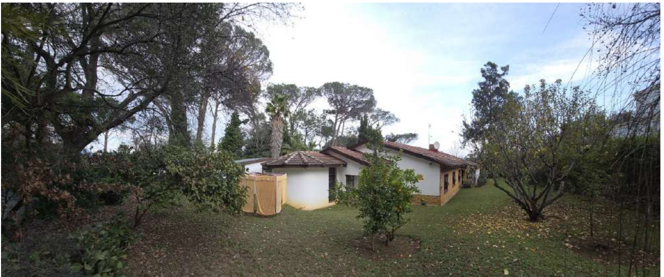
Figure 2: Eastern elevation of the dwelling on erf 5115, Stellenbosch.
