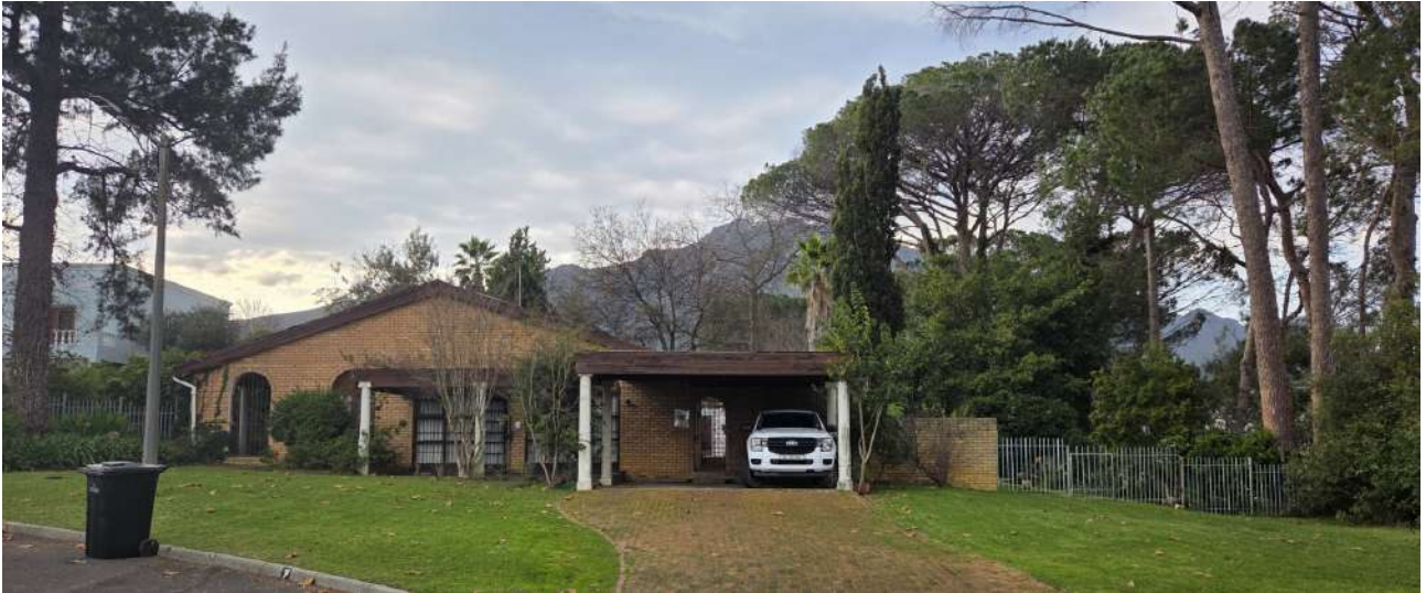
Figure 1: Street elevation of the dwelling on erf 5115, Stellenbosch.
