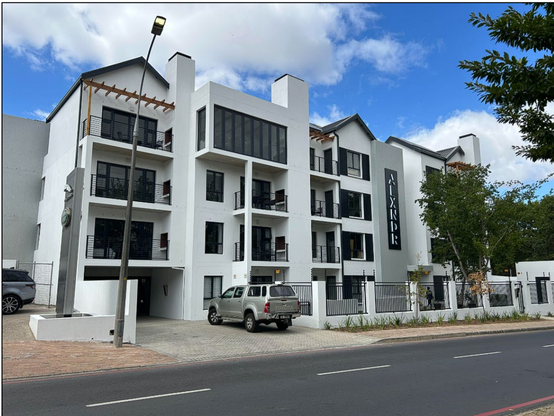
Figure 10 - Street Photo of Newly Constructed The Alxnder Building on Erf 263, Stellenbosch
