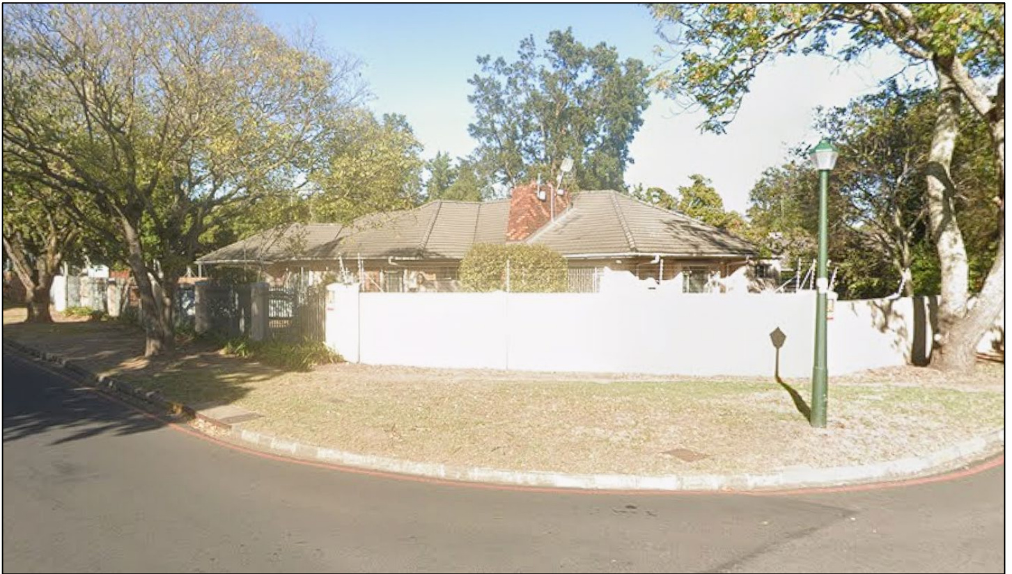
Figure 6 - Existing House from c/o Bergzicht Road and Du Toit Street
