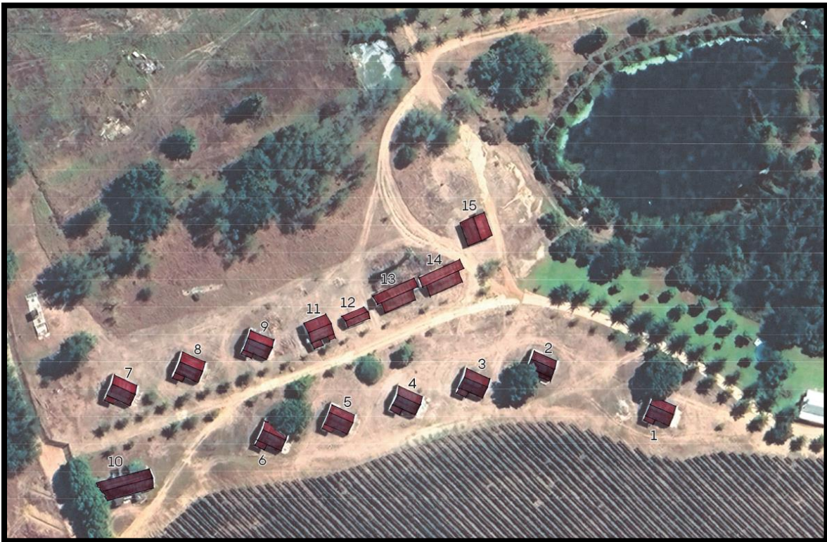
Figure 12 - 15 existing labourers' cottages
