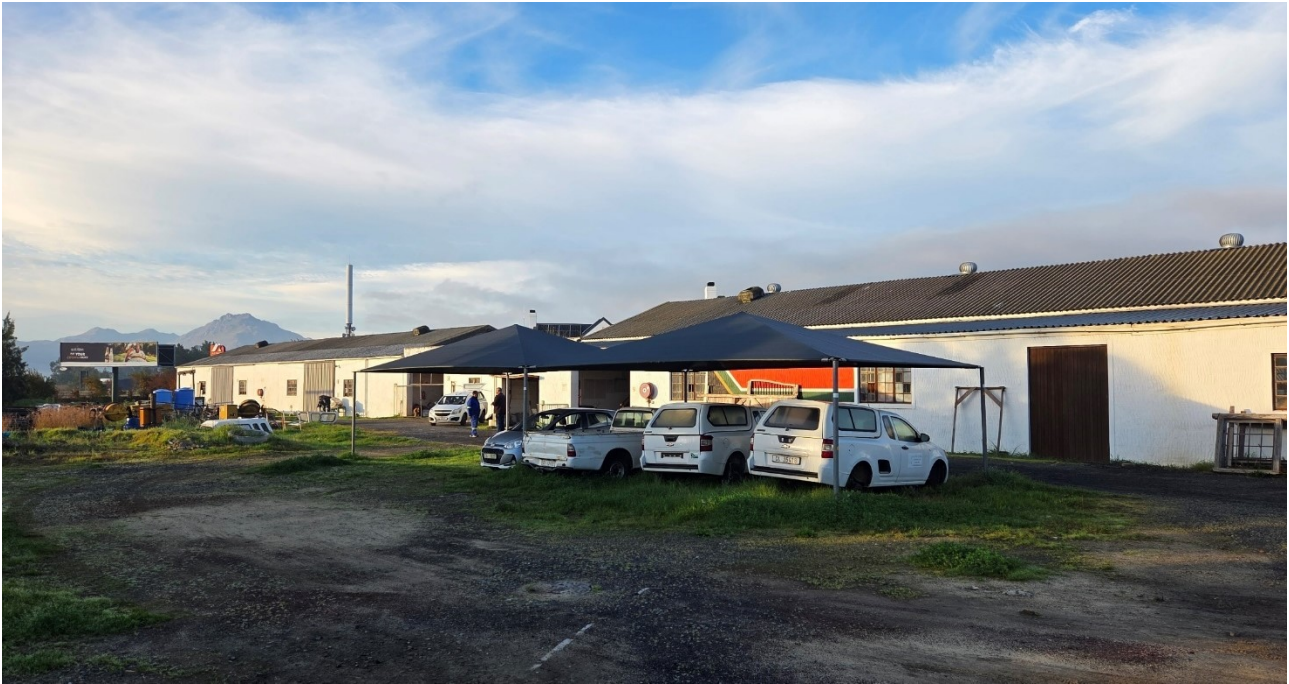
Figure 2: Photo of the existing store buildings associated with the builders' yard.
