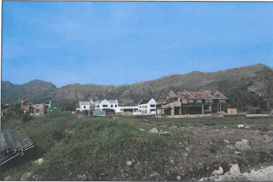
Photo 5 New development to the south
