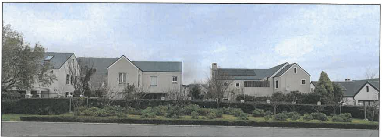
Photo 3 Example of Grouphousing complex in Kylemore
