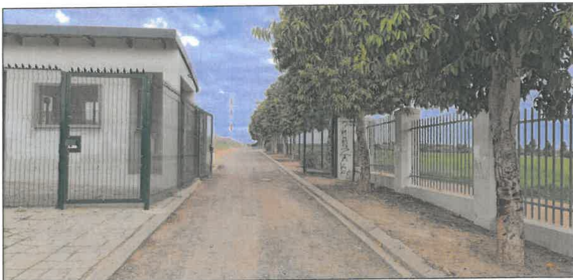
Figure 3: Photo of Existing Access Point of the Subject Property to/from School Street
