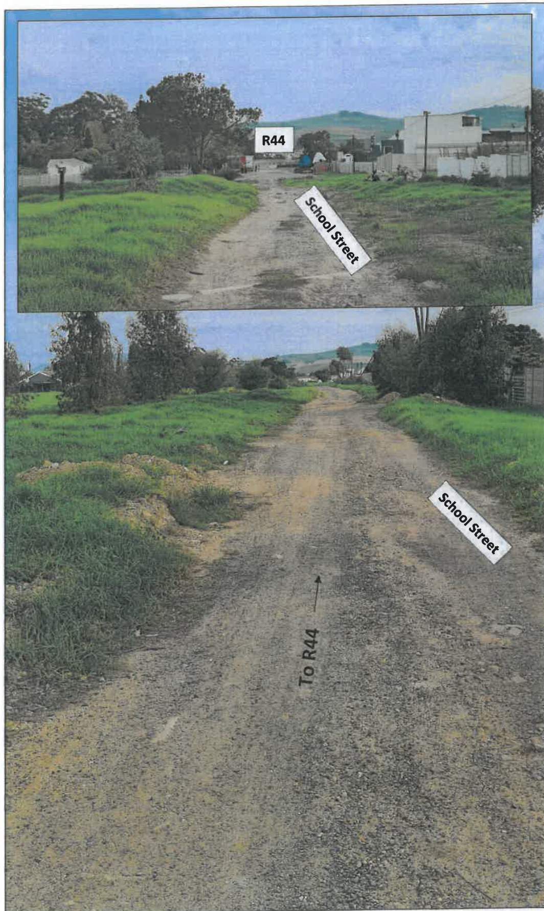
Figure 4: Current Condition of School Street between Blakemore Street and the Subject Property (Jamestown Sports Ground)
