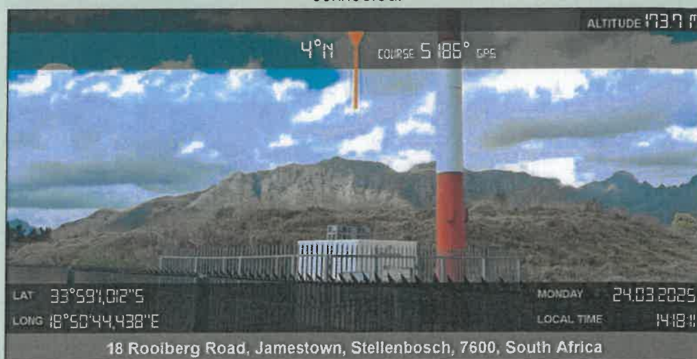
Figure 2: The site pictured from just beyond its southwestern corner. The Telkom tower and fenced-in infrastructure is seen. Just beyond this, the elevation of the site is apparent in comparison to the surrounding ground level.
