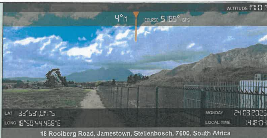
Figure 1: The gravel road alongside the site's western fence line. This gravel road is proposed to be the future access road for the fire station and will house future bulk service infrastructure to which the fire station will be connected.
