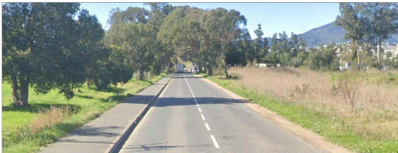
Figure 5: Kromme Rhee Road Eastbound
