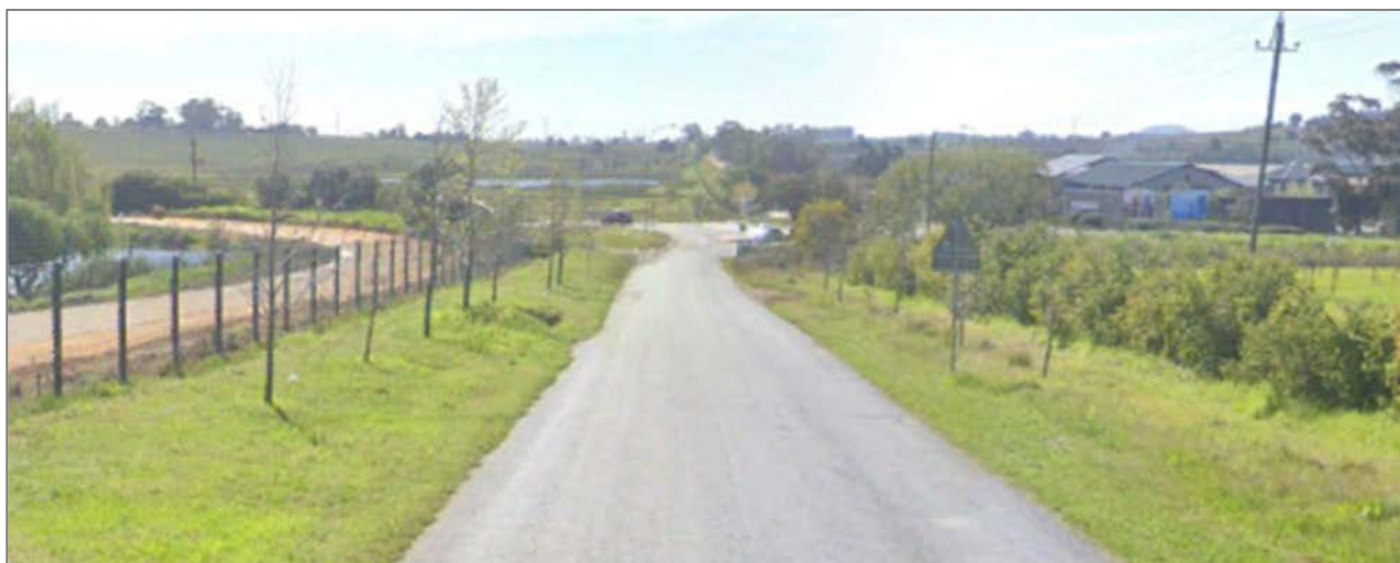
Figure 6: Blumberg Drive Northbound
