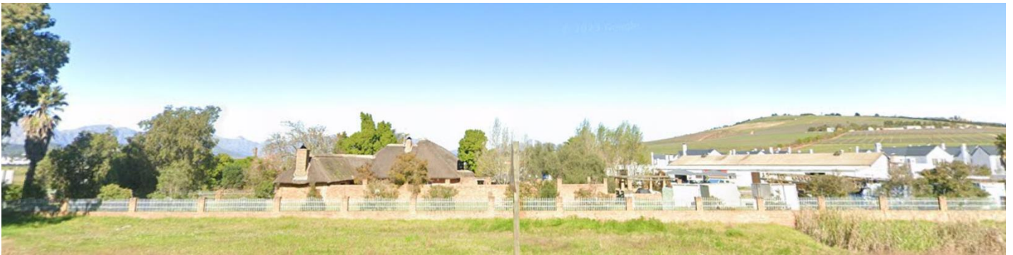
Photograph 13: the Basil Williams site at the intersection of the R304 and Bottelary Road (Source: Google Streetview)
