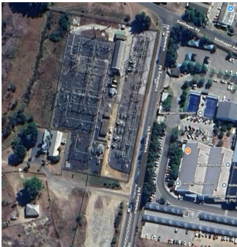
Stellenbosch Substation, Vredenburg road, Stellenbosch.
