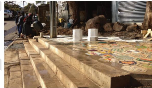
A washstand in Imizamo Yethu, Cape Town (Source: (Source: ArchSA, Issue 59, 2013)
