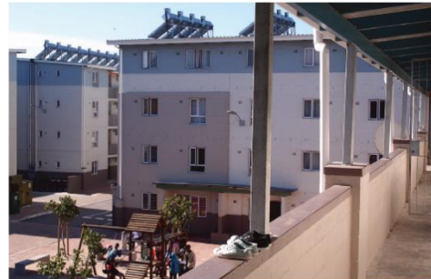
Community Residential Units, Langa, Cape Town (Source: Development Action Group)
