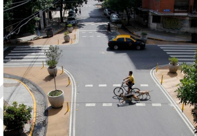
Crossing distance is reduced through painting, bollards and street trees (Source: Hampton for the University of Oklahoma, 2017)
