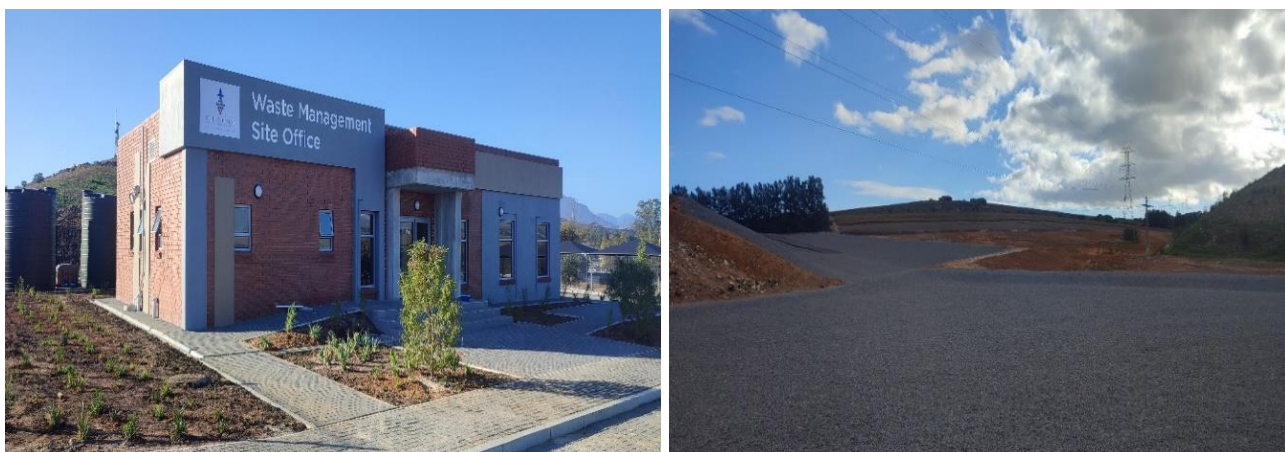
Image 20: Stellenbosch Landfill - Construction of New Assets
