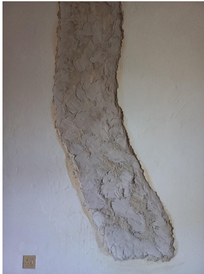
Figure 16 Wall repair in process
