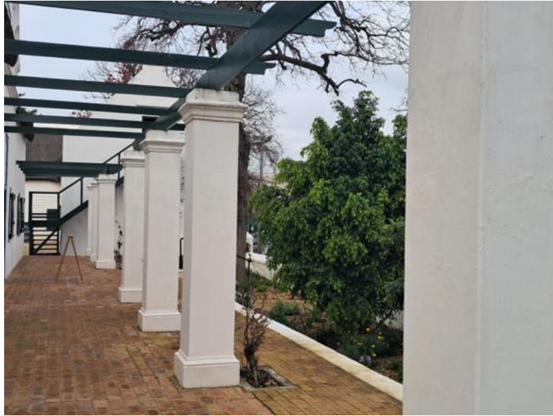
Figure 50 – Pergola's timber replacement.
