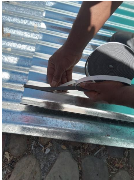
Figure 22. Installation of adhesive sealing strips
