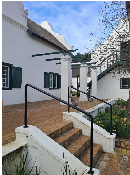
Figure 51 Minimal design balustrade added to the steps.
