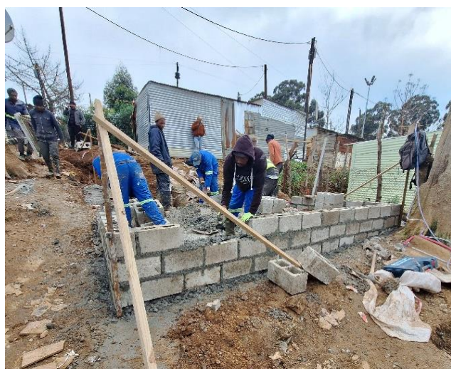
Image 7: Construction of ablution facilities in Enkanini, Kayamandi
