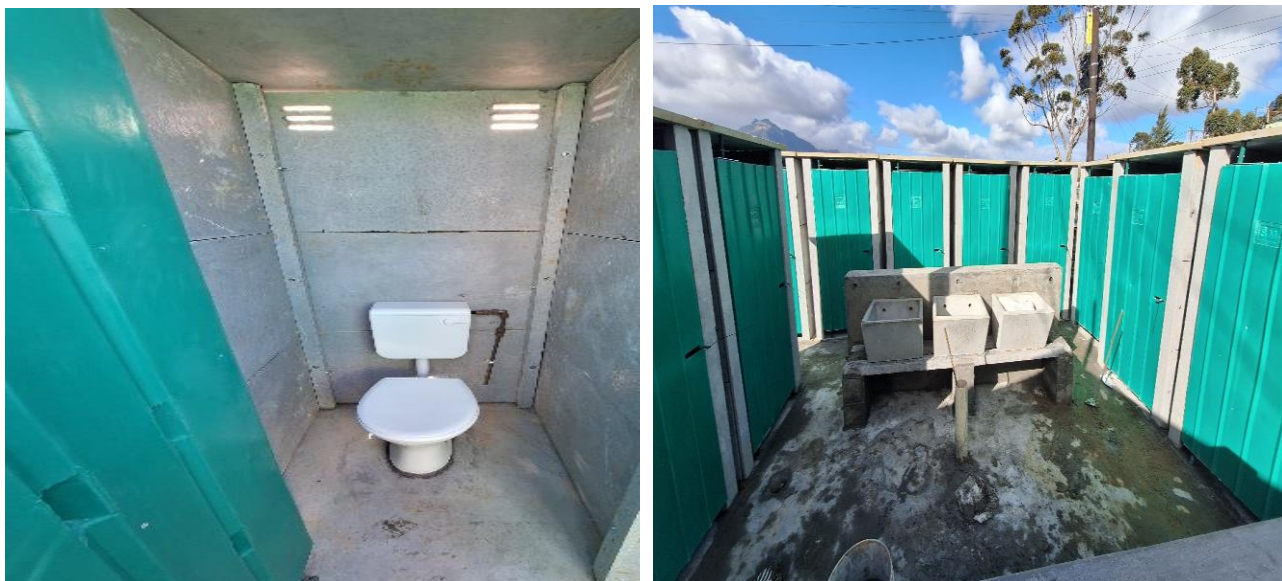
Image 8: Completion of ablution facilities
