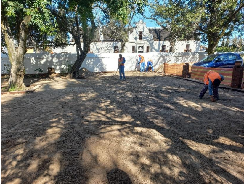
Figure 36 spreading the new sub-base
