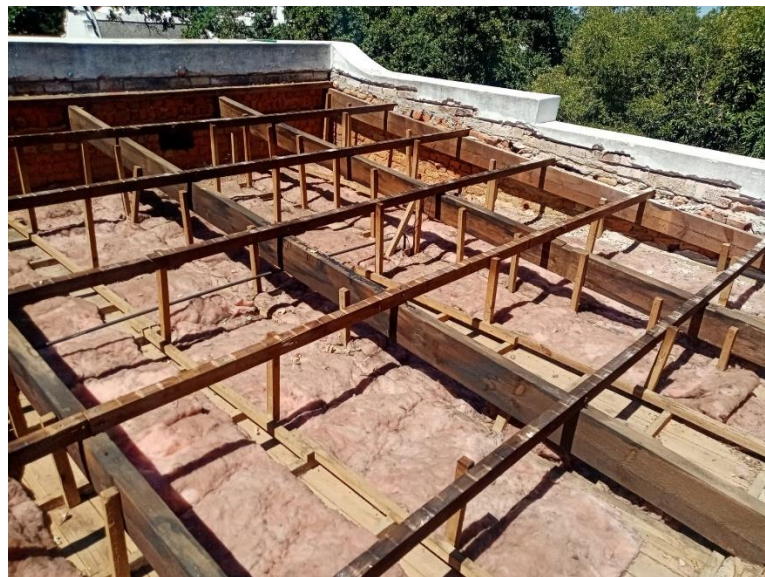
Figure 19 Existing timber structure proved to be in good condition, few battens needed replacement.
