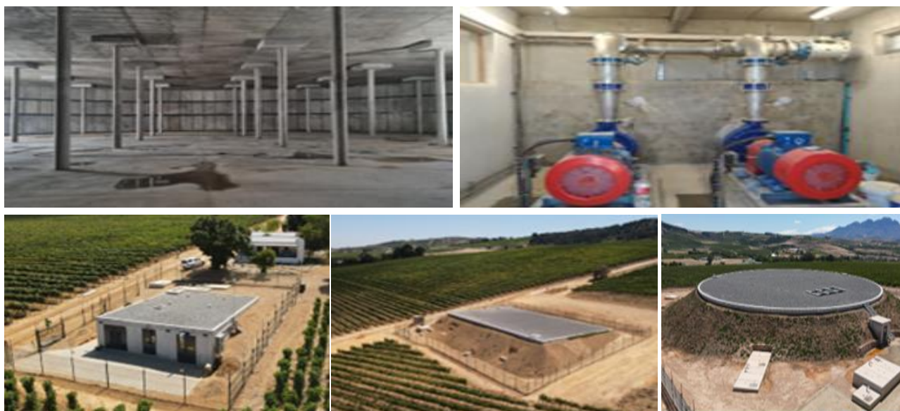
Image 17: Vloffenburg New Reservoir and Pipeline
