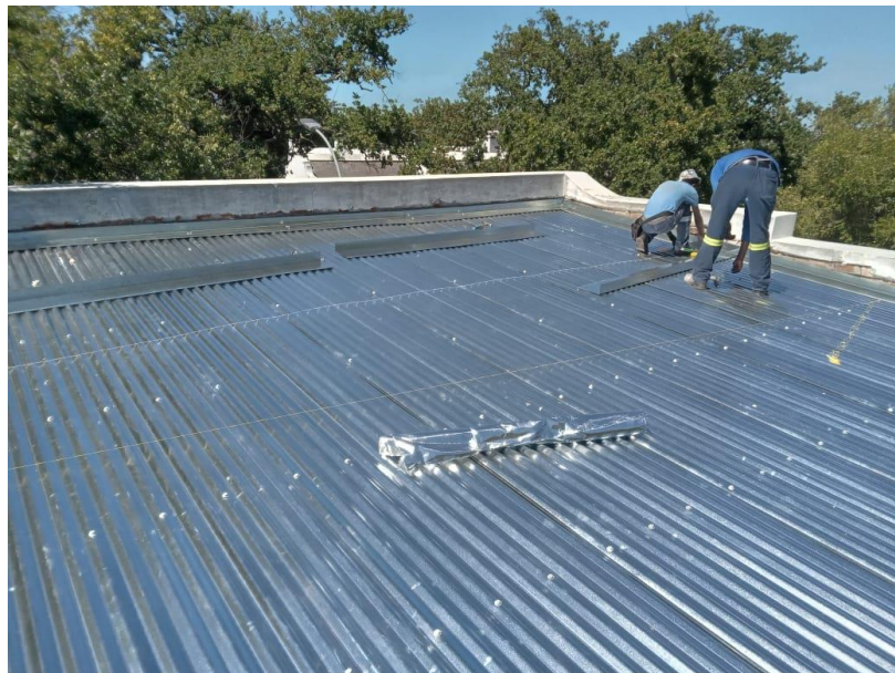
Figure 21. New corrugated roof sheeting
