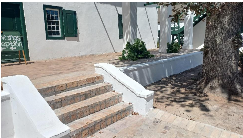
Figure 49 after the repair work
