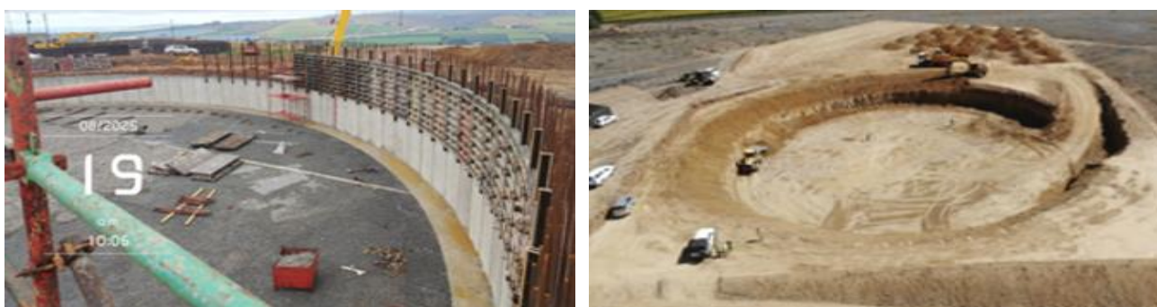
Image 19: Construction progress of the Stellenbosch 10ml Reservoir, Bulk Water Supply, and Associated Works
