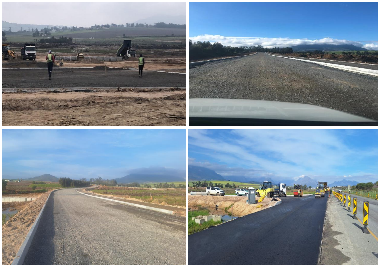
Image 14: Construction phase and access road of the Calcutta Memorial Park
