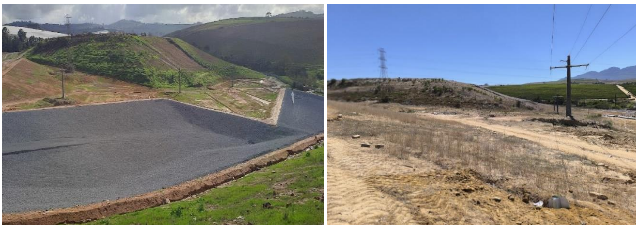
Image 21: Stellenbosch Landfill - Phase 2
