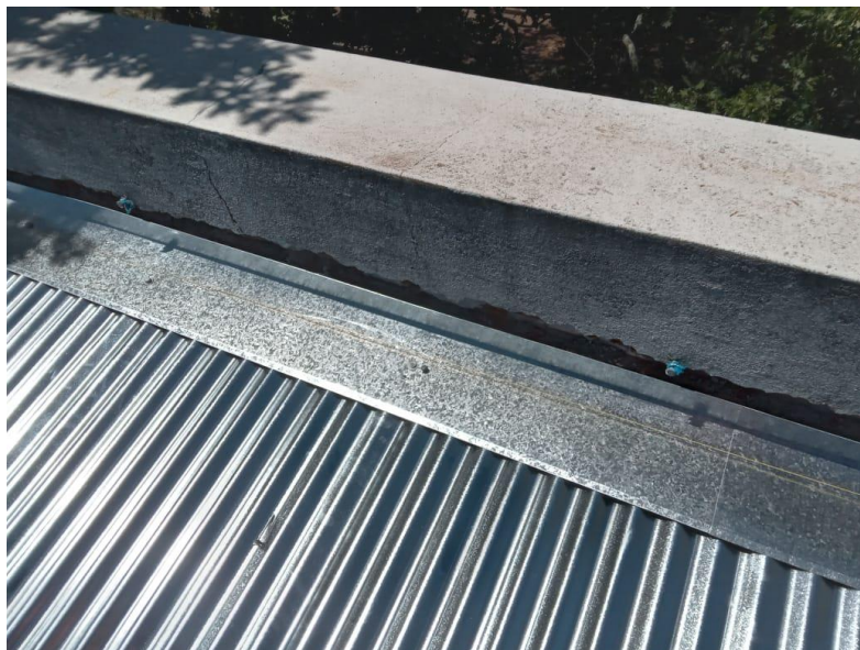
Figure 23. Metal flashings installation
