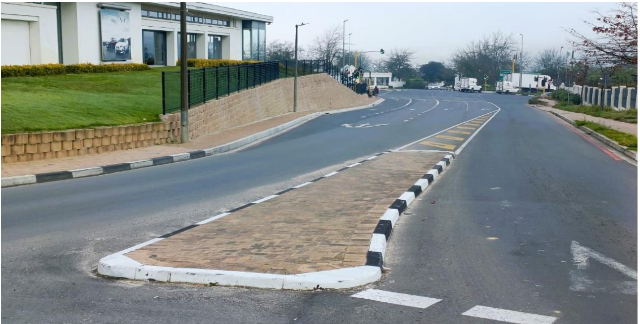
Image 27: R44 / Webersvallei Road Dedicated left turn lane (Jamestown)
