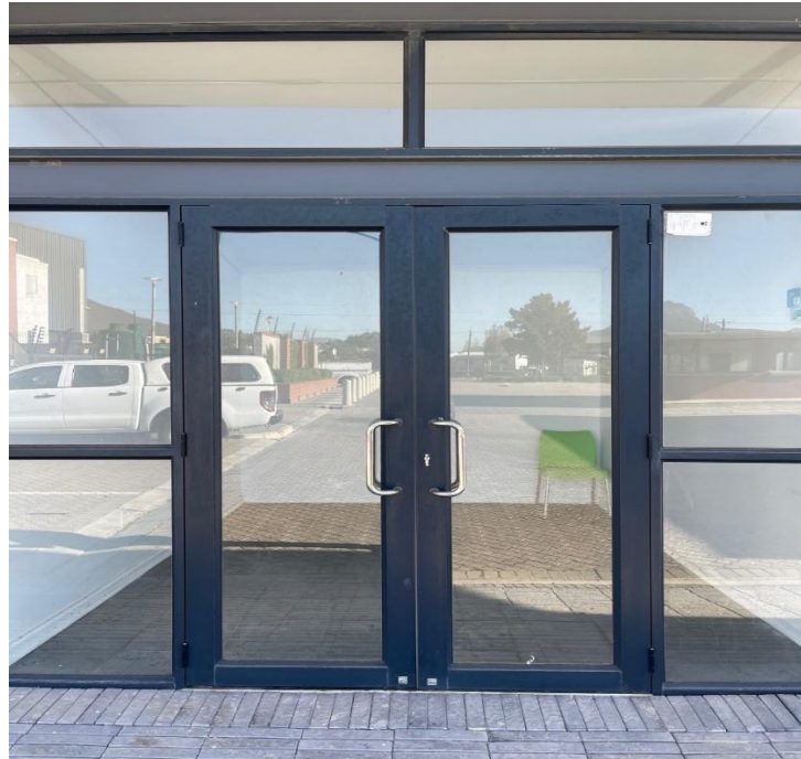
Vacant informal trading unit at the Klapmuts Informal Trading Hubs
