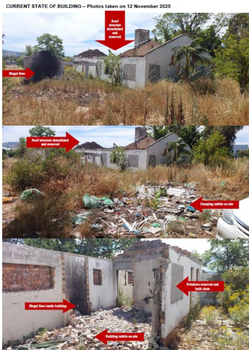
Figure 1: Current State of the structure
