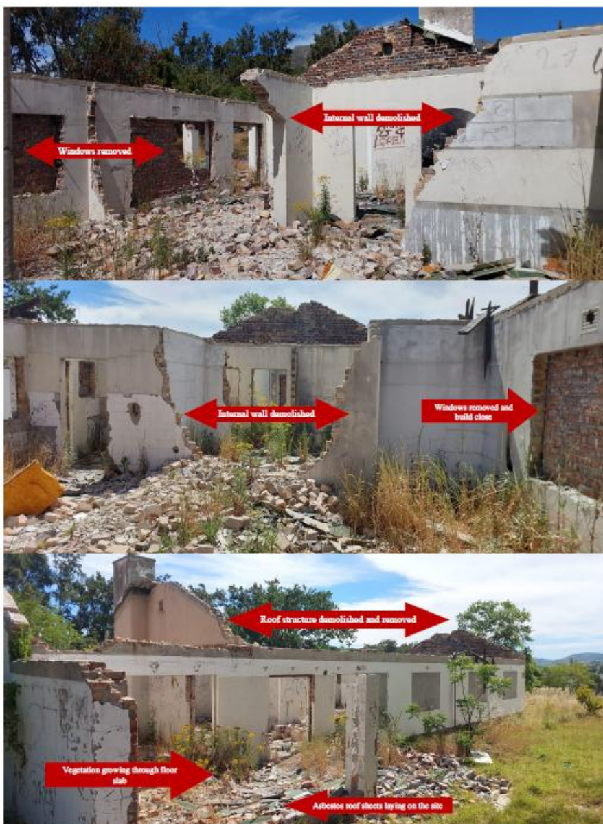
Figure 2: Current State of the structure
