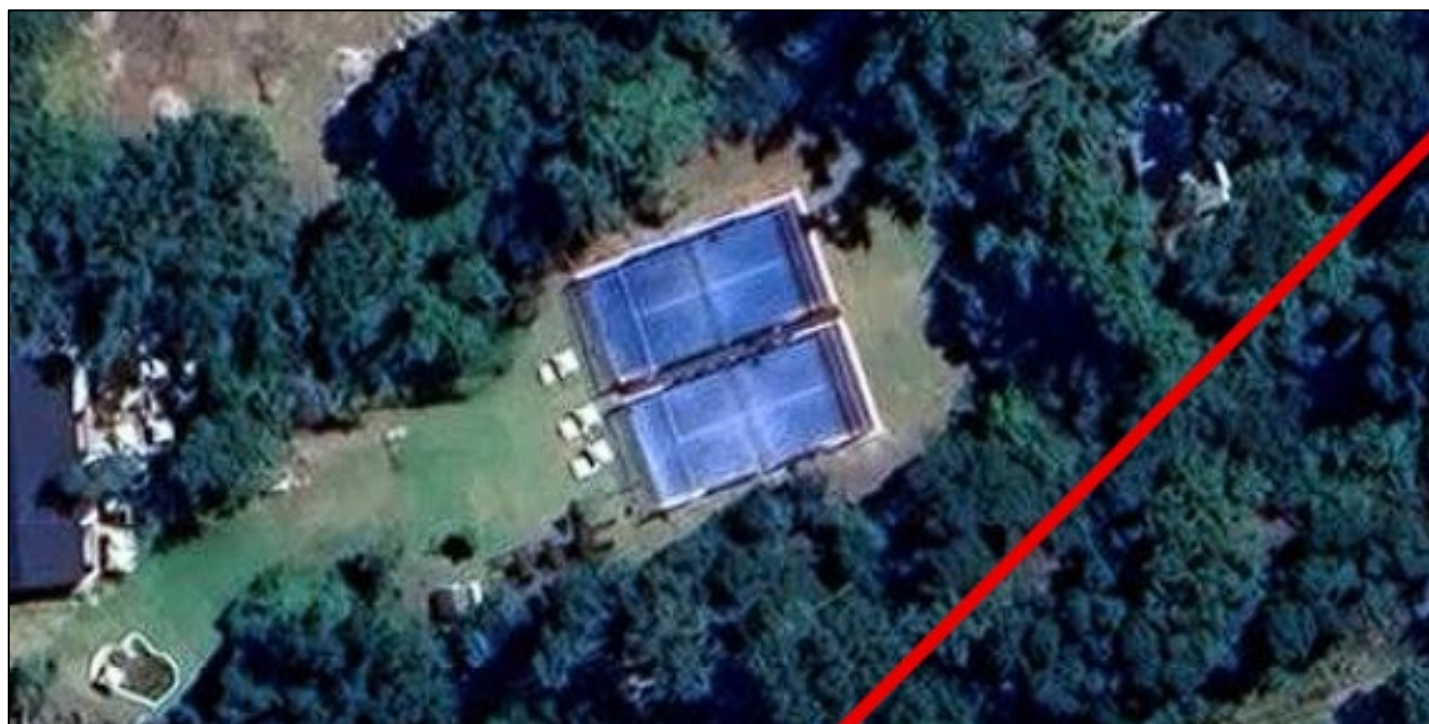
Figure 4 - Aerial Photo of Padel Courts
