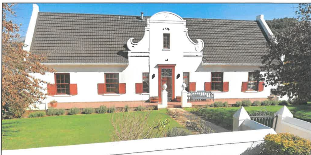
Figure 2: The existing dwelling house on Erf 74, Franschhoek
