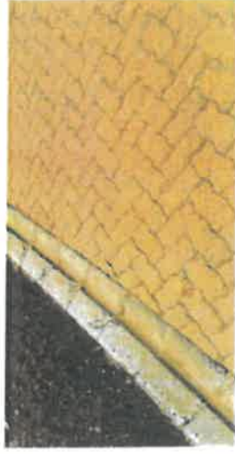
Figure 20 – road surface paving
