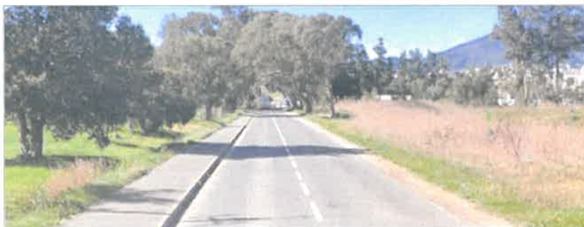
Figure 5: Kromme Rhee Road Eastbound
