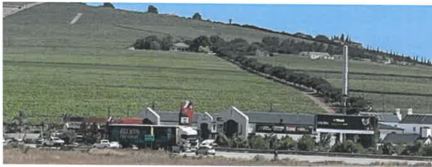
Photograph 10: The service station and commercial development to the south-west of the intersection (Sonop farm is visible against the hill behind)
