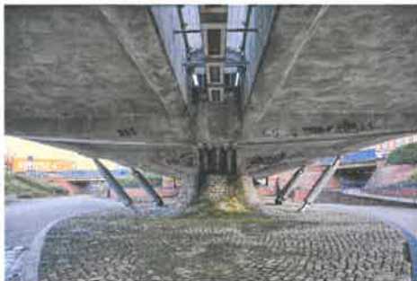
An elevated intersection with pedestrian access underneath
