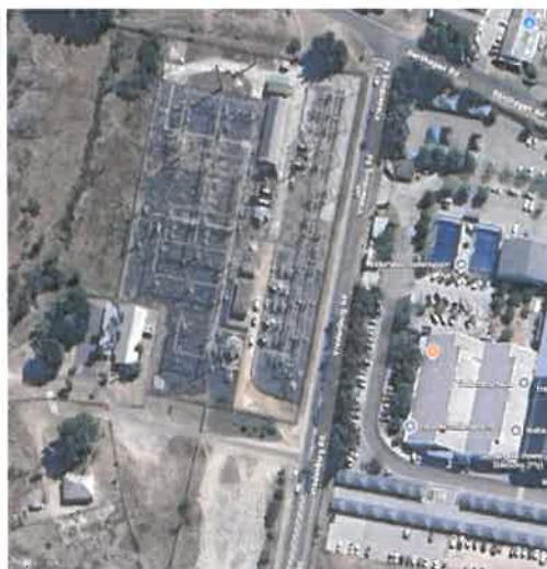
Stellenbosch Substation, Vredenburg road, Stellenbosch.
