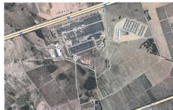
Muldersvlei Substation adjacent to the N1, in Klappmuts.
