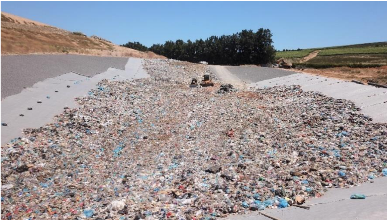
Image 5: Cell 4A at the landfill site
