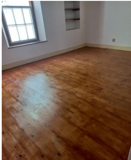
Figure 5 – timber tinting in process
