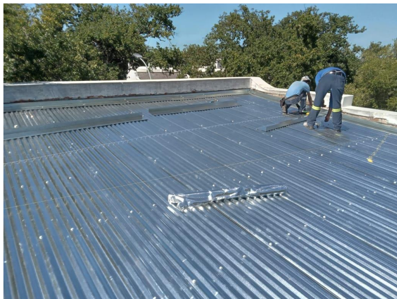
Figure 21. New corrugated roof sheeting
