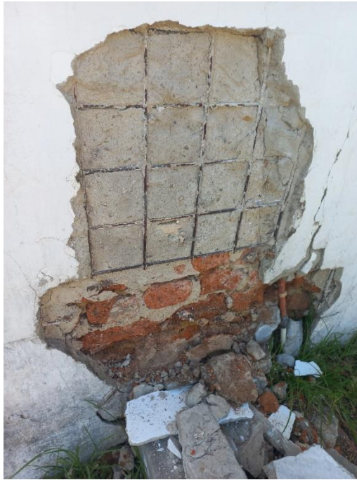
Figure 36 plaster delamination
