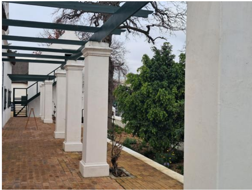
Figure 50 – Pergola's timber replacement.
