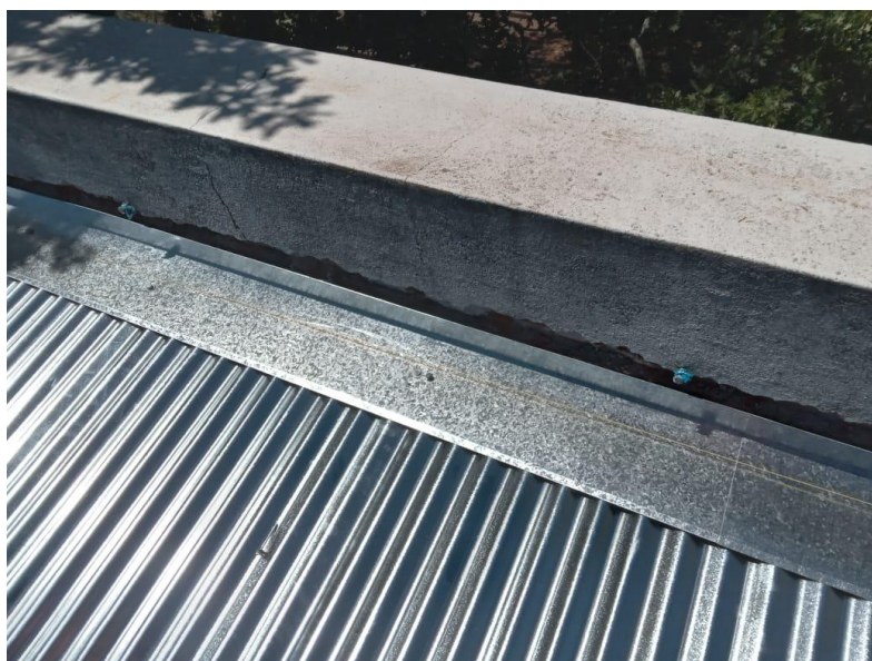
Figure 23. Metal flashings installation
