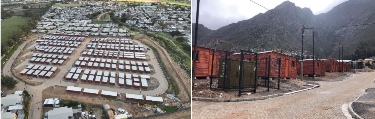
Image 12: Erf 3229: Mooiwater - Dam Rehabilitation and TRA Franschhoek
