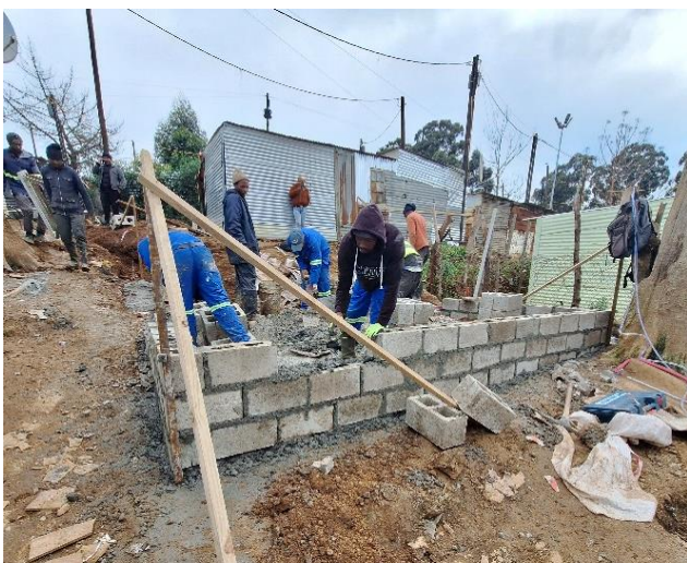
Image 7: Construction of ablution facilities in Enkanini, Kayamandi
