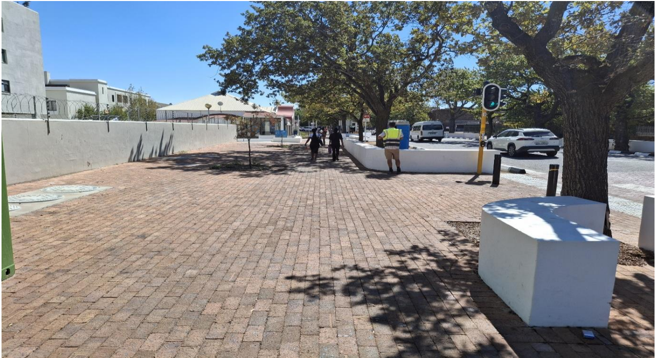
Image 11: External improvements to Bird Street and the implementation of pedestrian crossings
