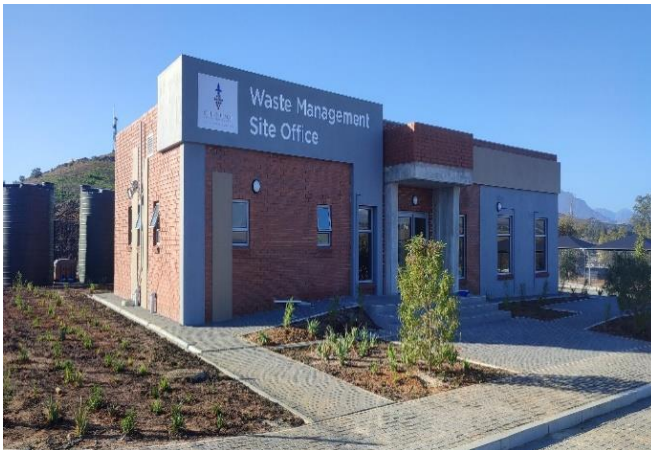
Image 20: Stellenbosch Landfill - Construction of New Assets
