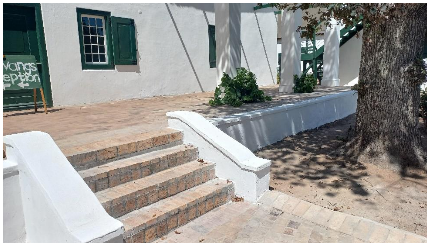
Figure 49 after the repair work
