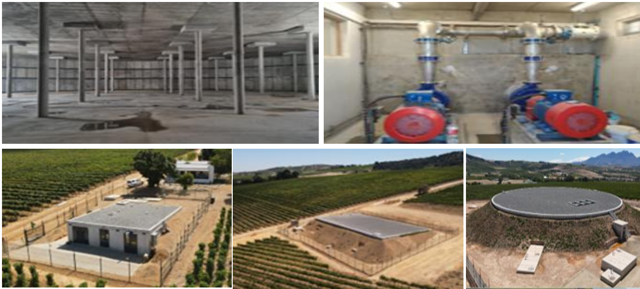
Image 17: Vloffenburg New Reservoir and Pipeline
