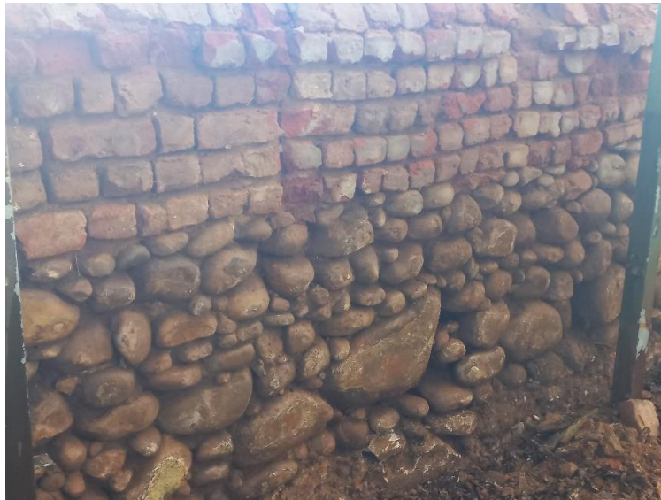
Figure 27 After the removal of the cement plaster
