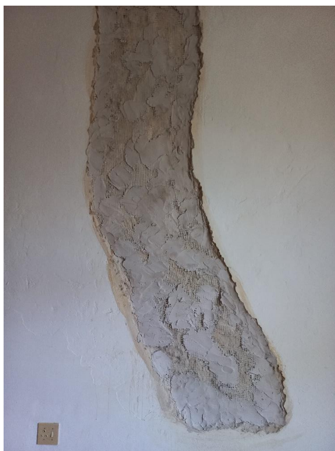
Figure 16 Wall repair in process
