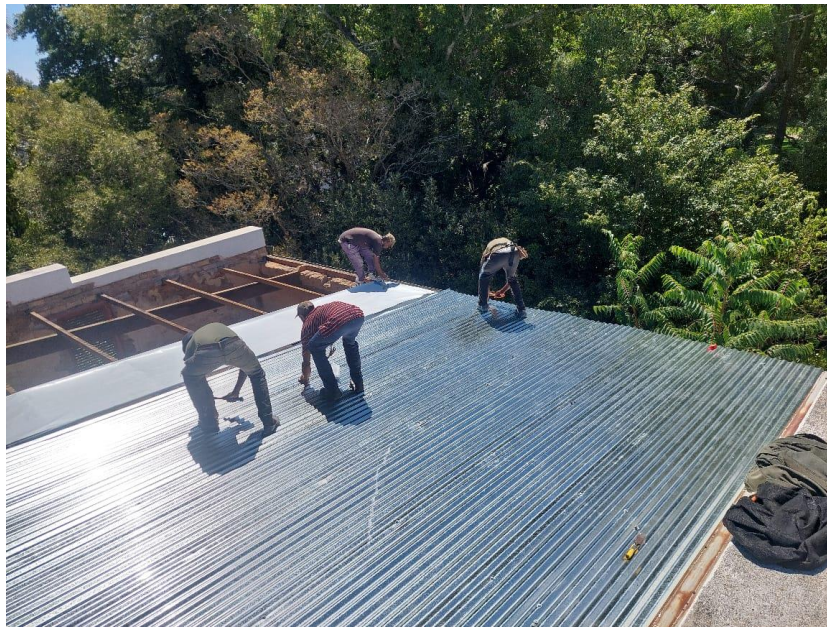
Figure 20. Under roof sheeting membrane installation
