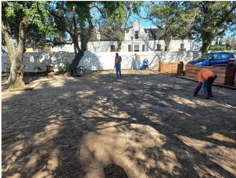
Figure 36 spreading the new sub-base
