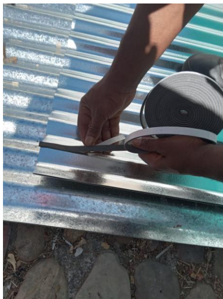
Figure 22. Installation of adhesive sealing strips
