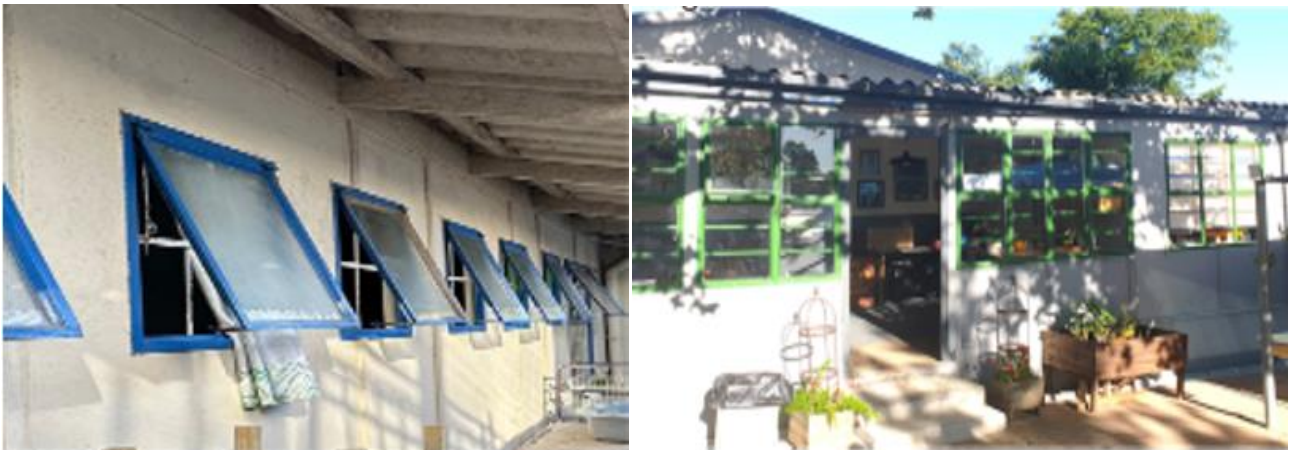
Image 13: Upgrading of Municipal ECD Facilities
