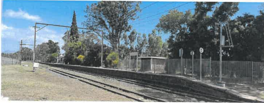
Photograph 9: The Koelenhof station as viewed from the Kromme Rhee Road railway crossing
