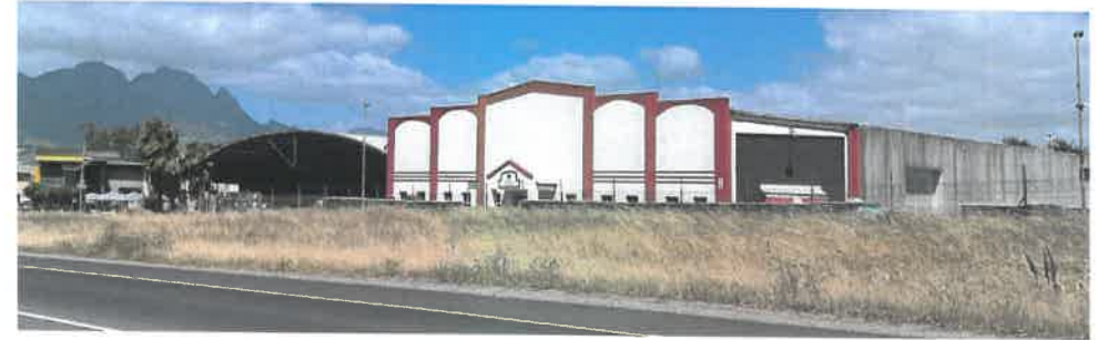
Photograph 12: Industrial development, to the west of Koelenbosch, as viewed from the Bottelary Road
