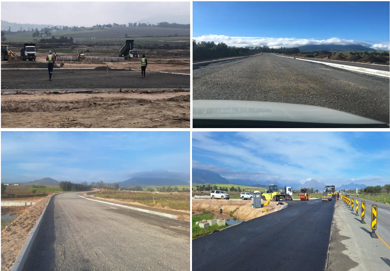
Image 17: Construction phase and access road of the Calcutta Memorial Park
