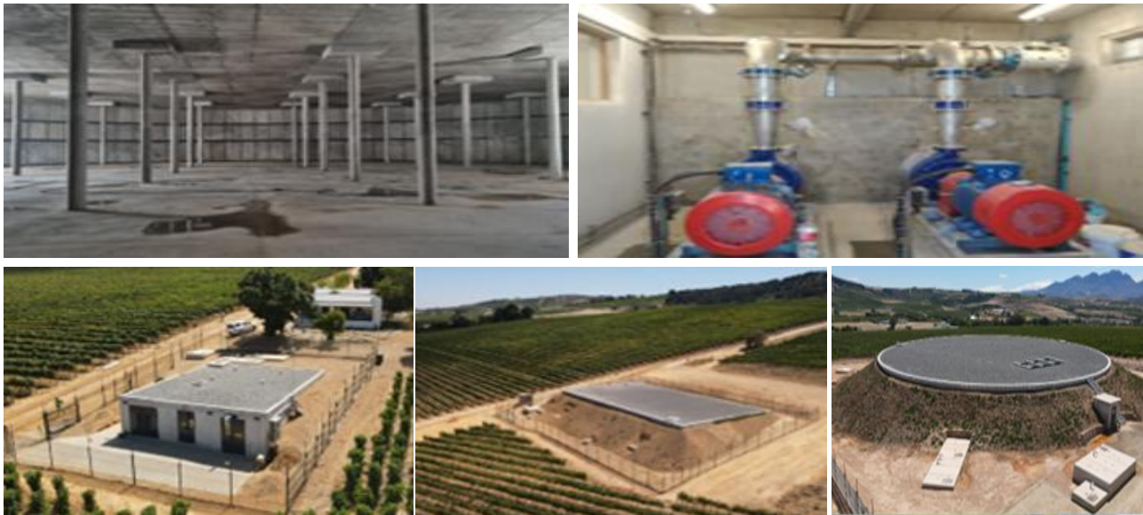
Image 19: Vloffenburg New Reservoir and Pipeline
