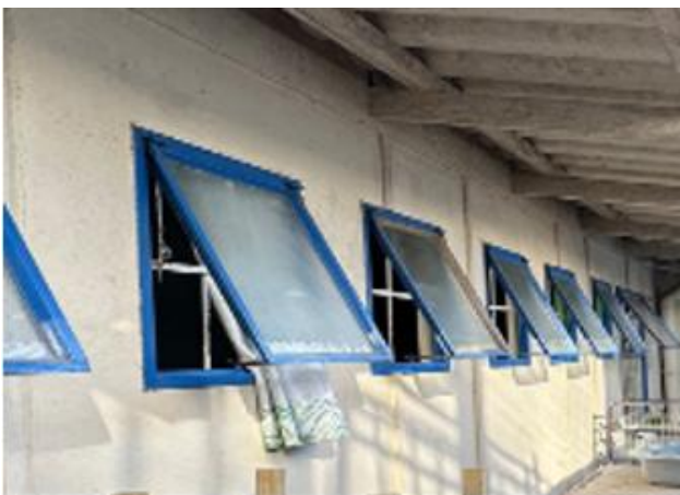
Image 16: Upgrading of Municipal ECD Facilities
