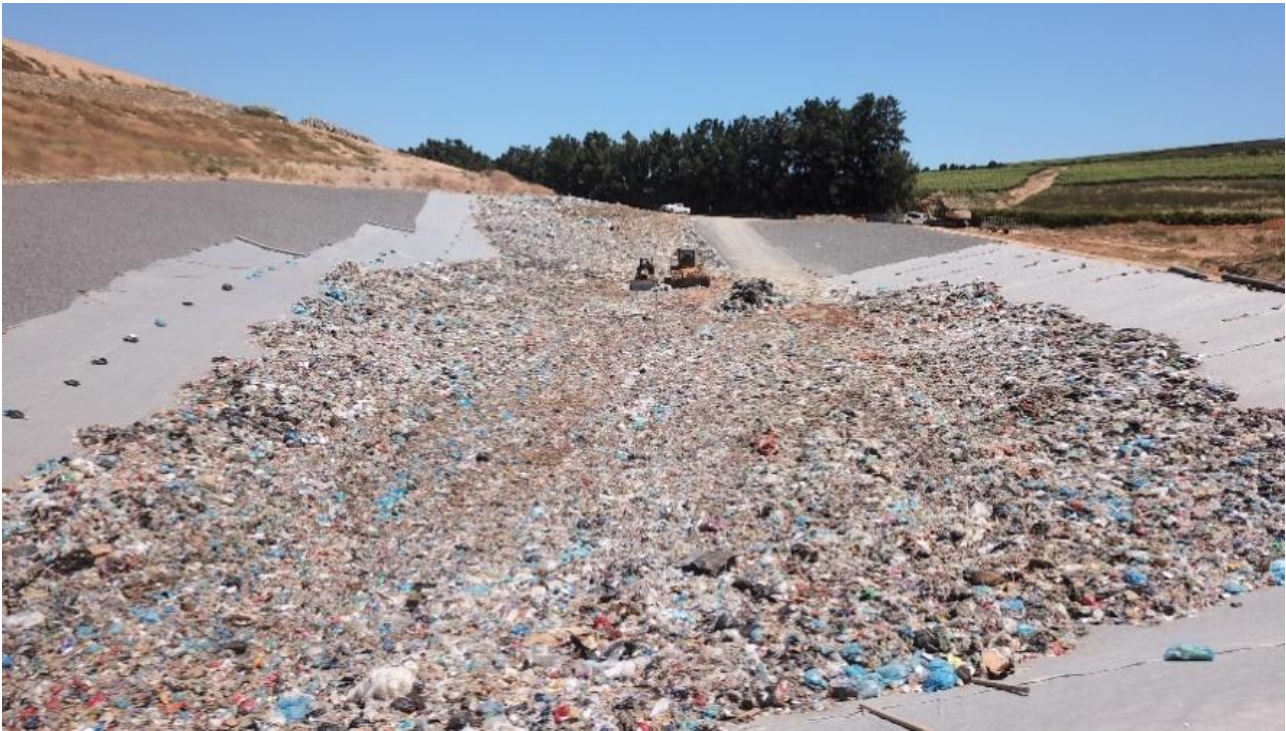
Image 5: Cell 4A at the landfill site
