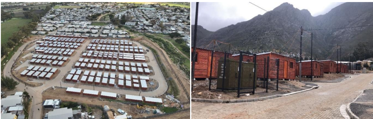
Image 15: Erf 3229: Mooiwater - Dam Rehabilitation and TRA Franschhoek
