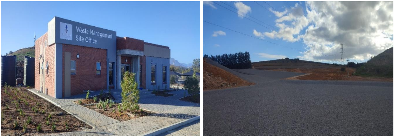
Image 21: Stellenbosch Landfill - Construction of New Assets
