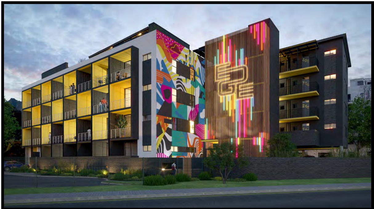
Figure 6: The Edge student flats on Erf 17349
