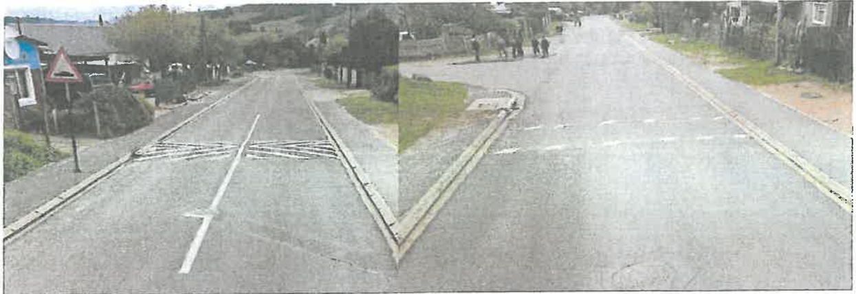
Speed hump along Skool Street
