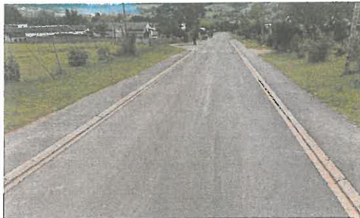
Sidewalks along both sides of Skool Street
