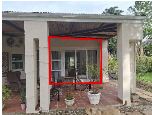
Figure 10: Enclosure of stoep area
