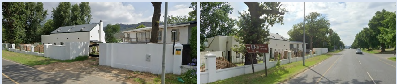
View from Main Road 191 (R45)
