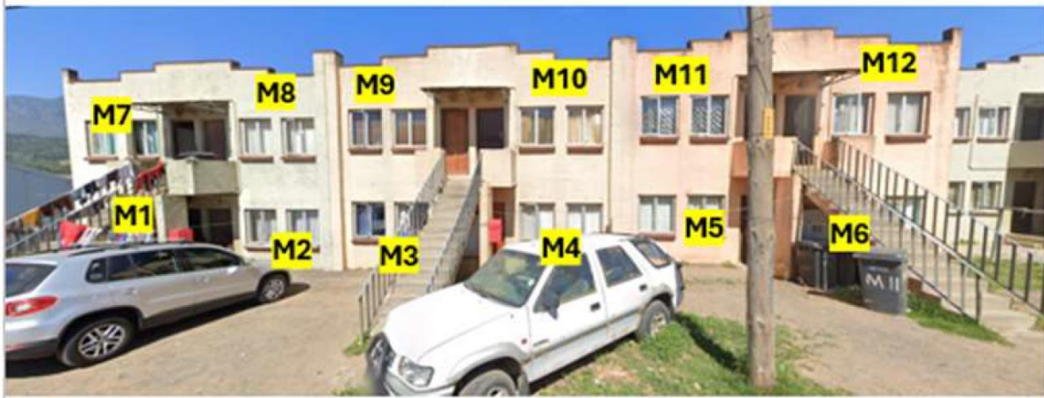
Figure 14: Block M Housing Units
