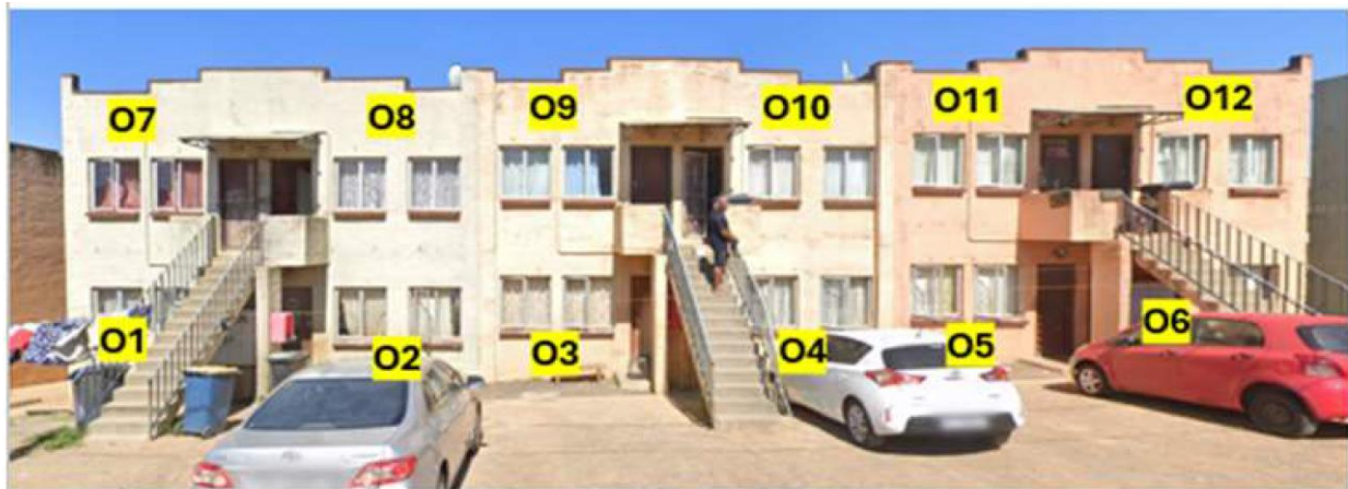
Figure 16: Block O Housing Units
