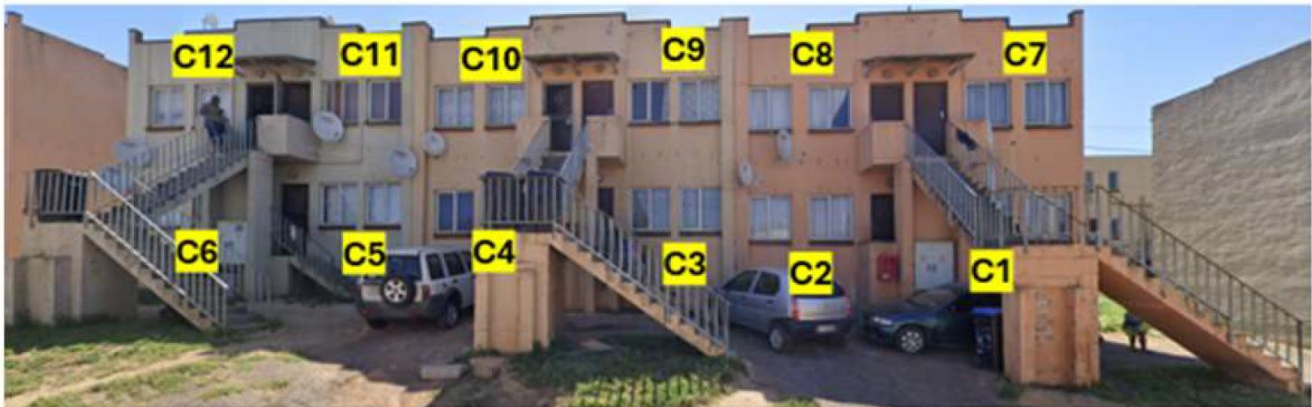
Figure 4: Block C Housing Units
