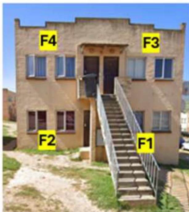
Figure 7: Block F Housing Units
