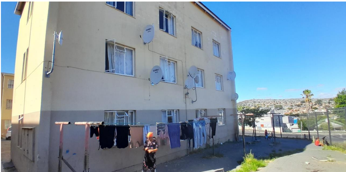
Fig 1: DSTV dishes to be removed & reinstalled
