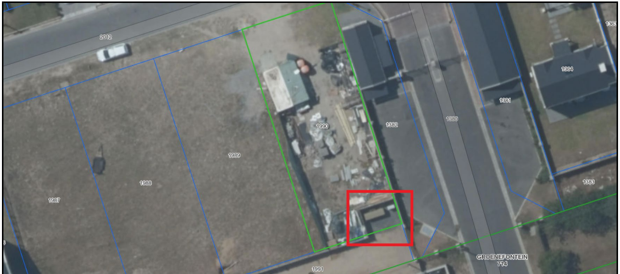
Figure 2: The electrical substation on Erf 1990, Klapmuts
