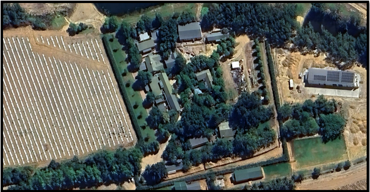
Figure 2: Buildings and structures on Farm 100/2, Stellenbosch
