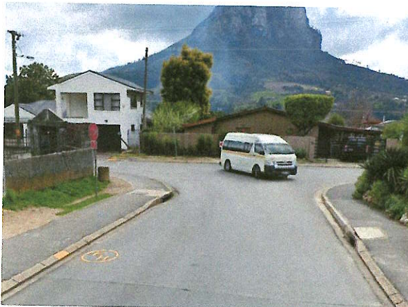
Skool Street/Brandt Street intersection
