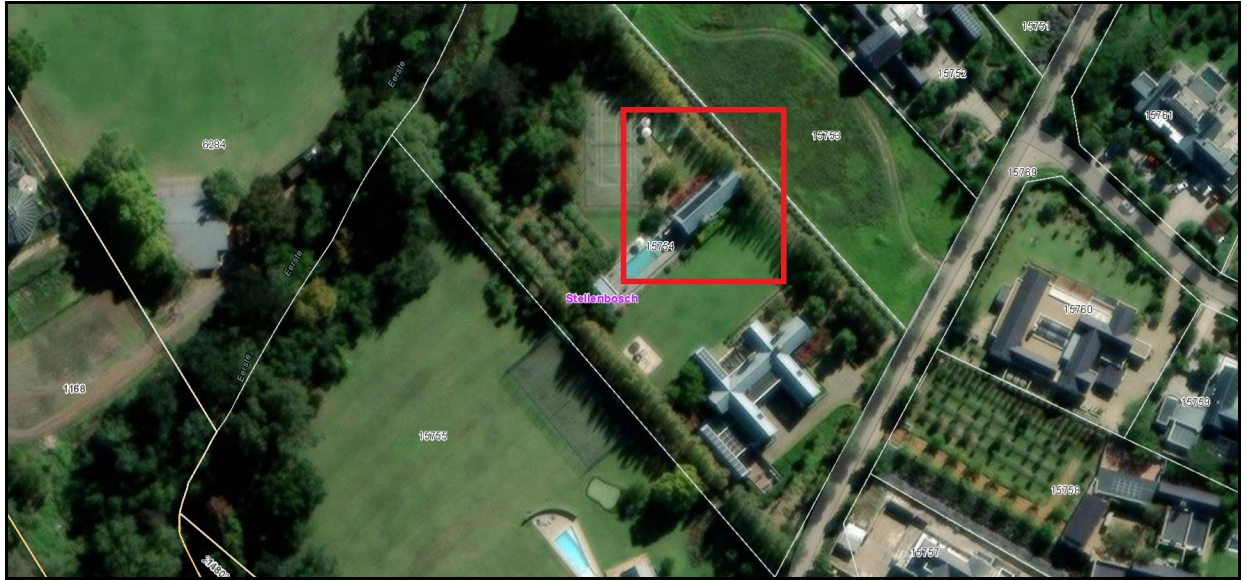
Figure 4: Pool house at De Bosch Erf 15754
