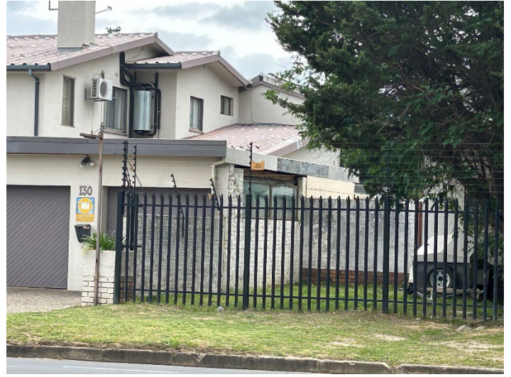
Figure 6 – Window on common boundary line of application site (built on the 0m boundary line), Erf 223
