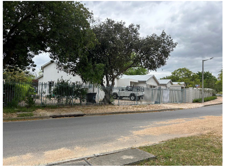
Figure 8 - Erf 2220, with second dwelling unit
