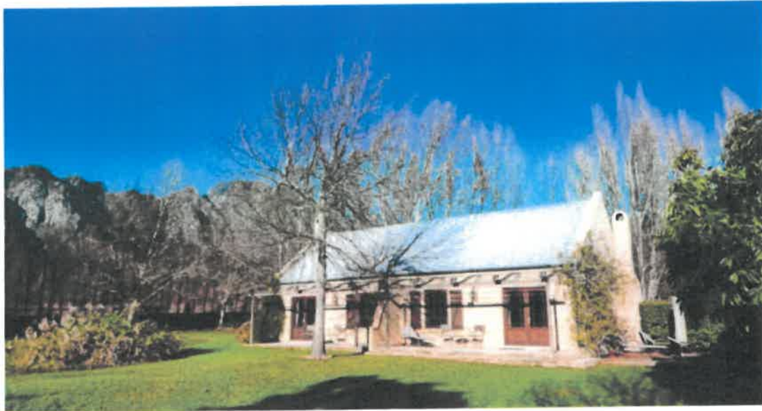
Figure 4: Present state of one of the cottages on site.
