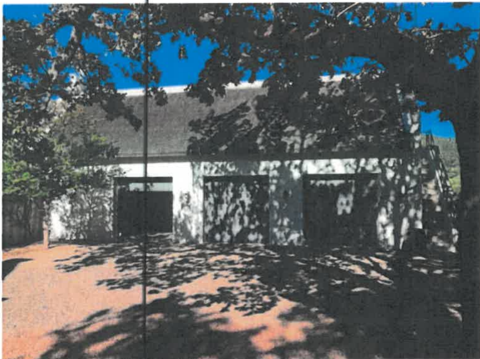
Existing triple garage building (subject of this application)
