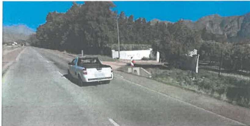
Figure 1-2 Central and Main Entrance from the R301
