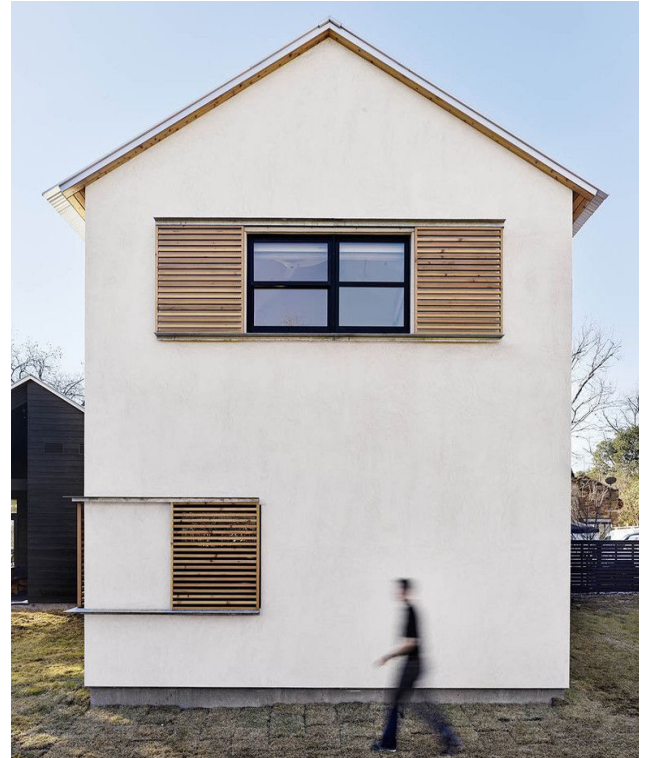
Figure 38: Timber sliding shutters
