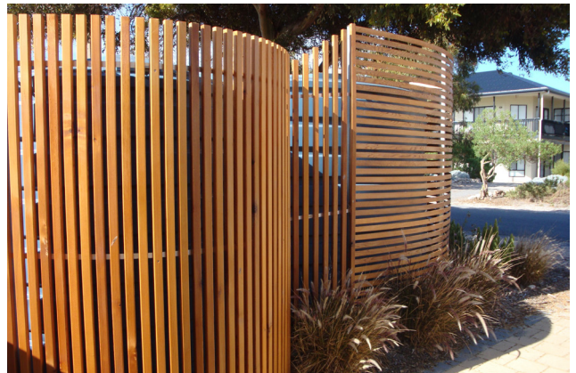
Figure 41: Timber slats used to conceal rainwater harvesting tanks
