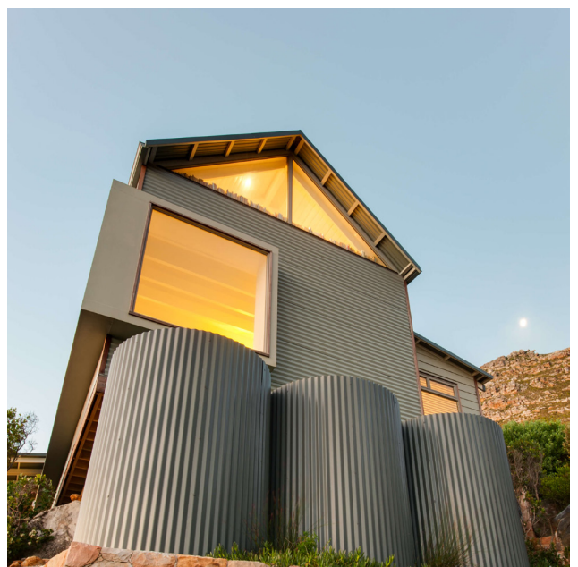
Figure 42: Metal cladding used to conceal rainwater tanks
