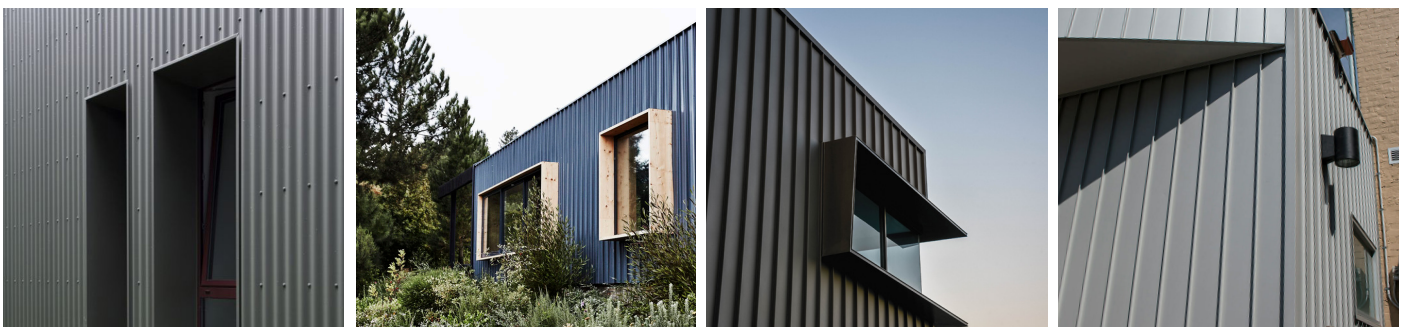
Figure 18: Sheet piling as side cladding examples.
