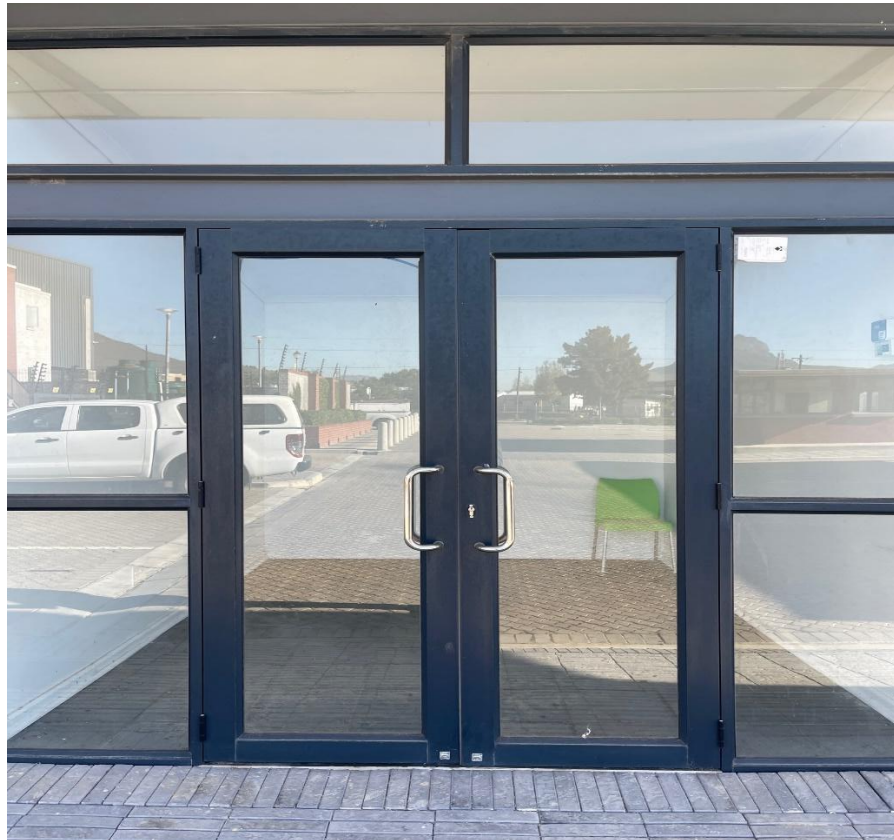
Vacant informal trading unit at the Klappmuts Informal Trading Hubs
