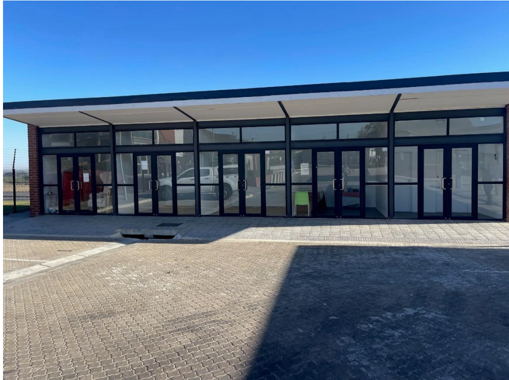
Vacant informal trading units at the Klapmuts Informal Trading Hubs
