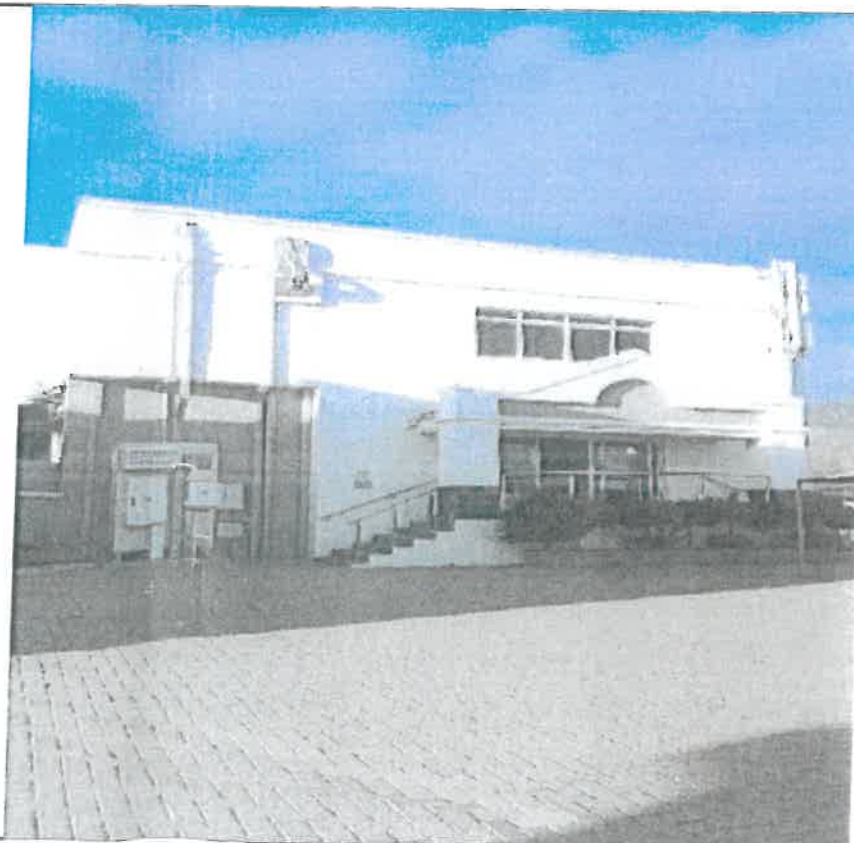
Existing rooftop site
