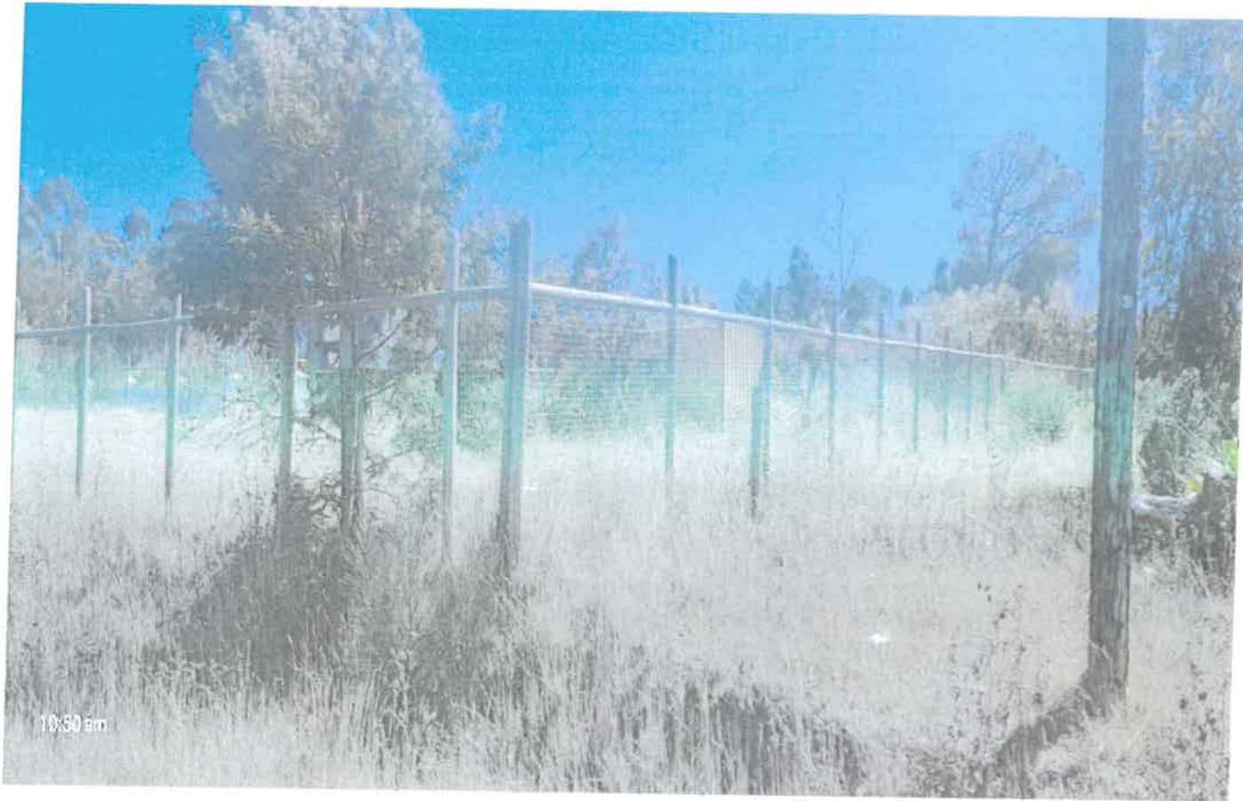
View of Erf 406RB from Minor Road
