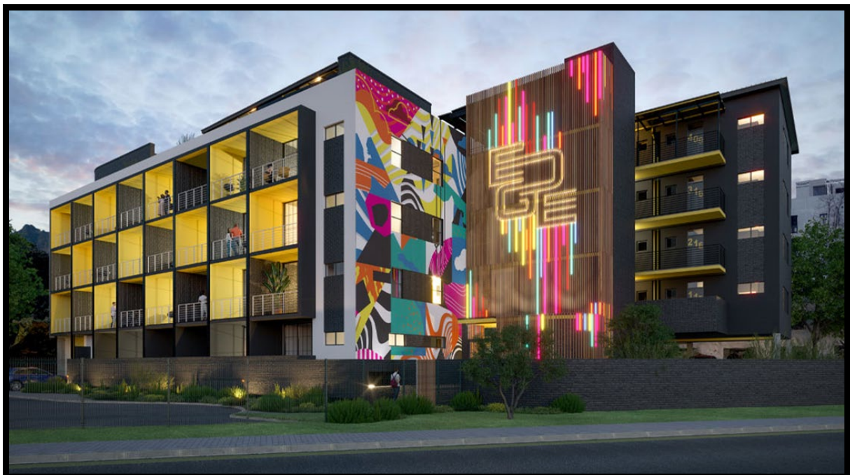
Figure 5: The Edge student flats on Erf 17349
