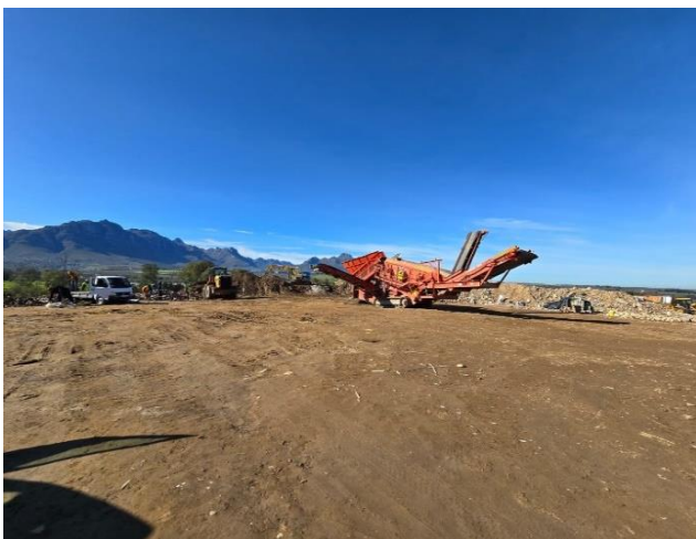
Crushing of builder's rubble
