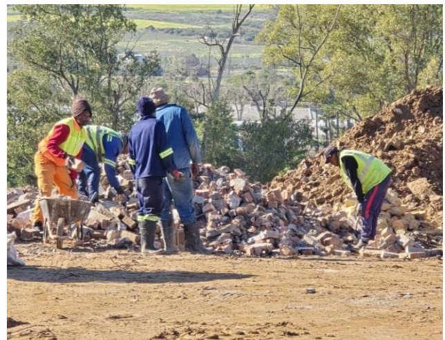
Reclaiming of bricks at the site
