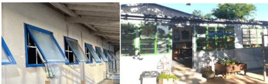
Upgrading of Municipal ECD facilities.
