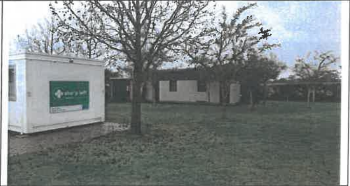
Skills centre adjacent to clinic
