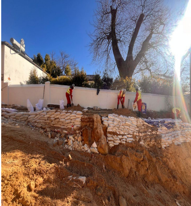
September 2024 - Sand bags support to boundary wall foundations and lateral support of embankments
