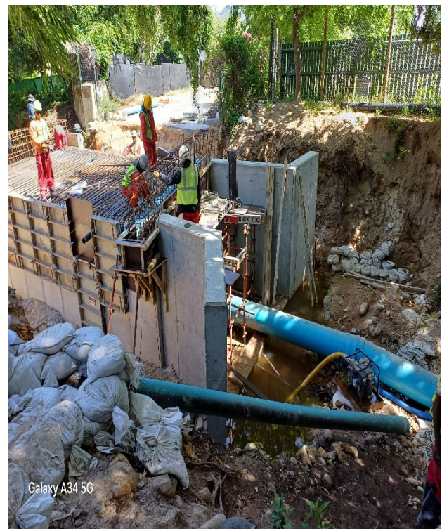
November 2024 - Construction of street culverts in Akademie Street
