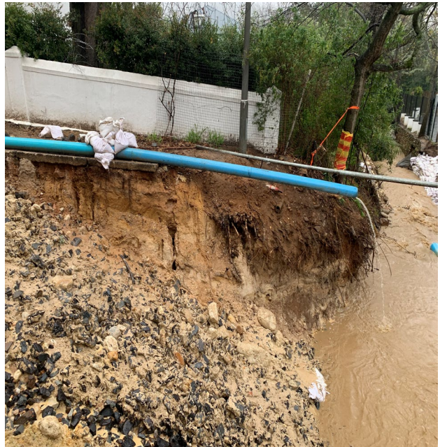
July 2024 - Eroded embankments after rainfall
