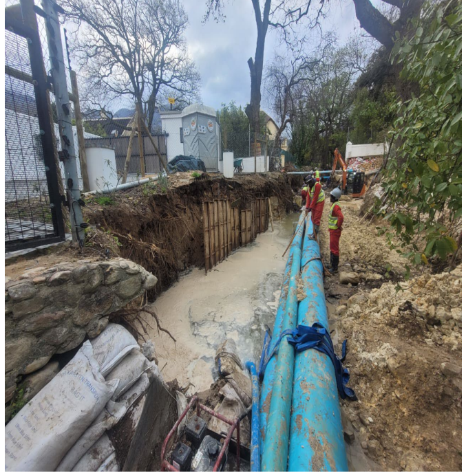
September 2024 - Sand bags support to boundary wall foundations and lateral support of embankments
