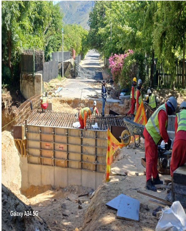
November 2024 - Construction of street culverts in Akademie Street
