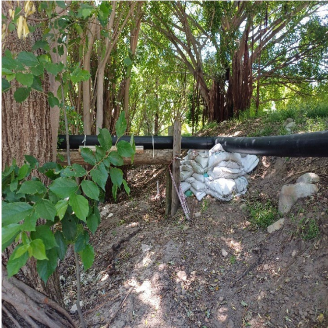
August 2024 - Temporary deviation of bulk watermain in Akademie Street
