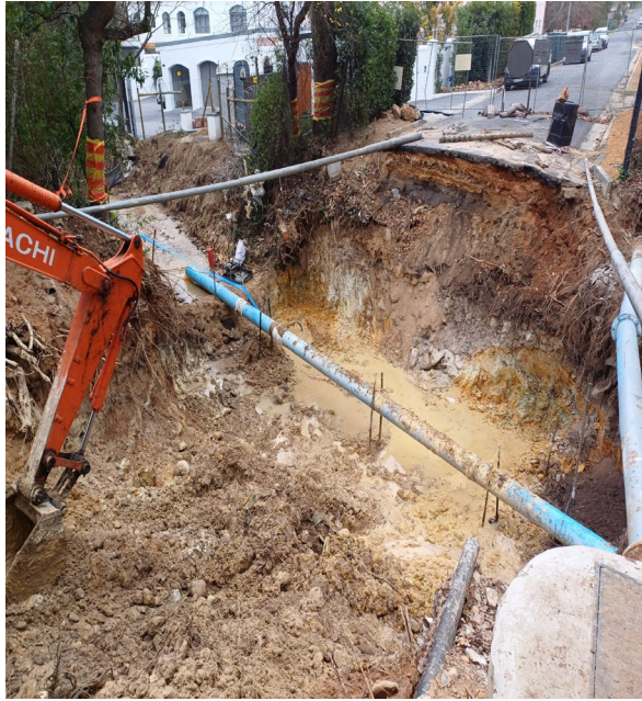
July 2024 - Eroded embankments after rainfall
