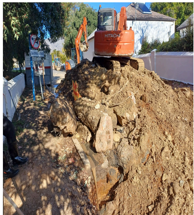
June 2024 - Intermediate excavation in saturated riverbed
