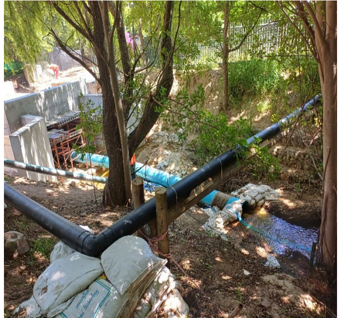
August 2024 - Temporary deviation of bulk watermain in Akademie Street
