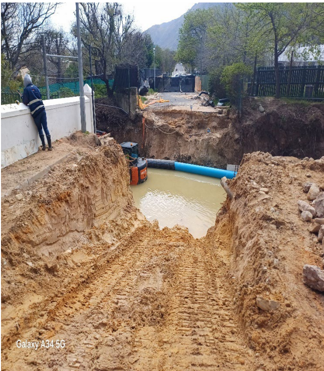
September 2024 - Reinstatement of construction ramp after the heavy rainfall
