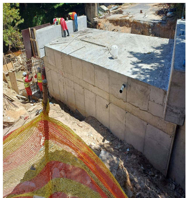
November 2024 - Construction of street culverts in Akademie Street Culvert
