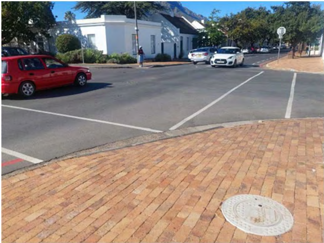
Figure 5-5: Unsafe orientation of dropped kerbs
