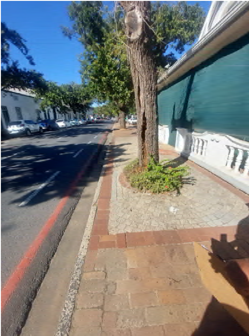
Figure 5-4: Obstructions in pedestrian walkways
