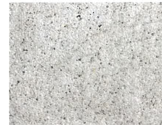
Exposed aggregate concrete
