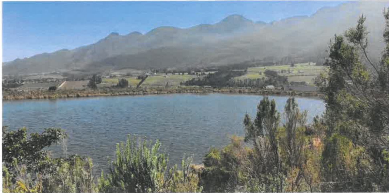
View across the dam
