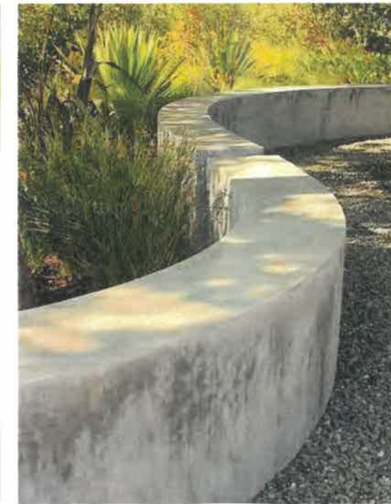
Low concrete walls
