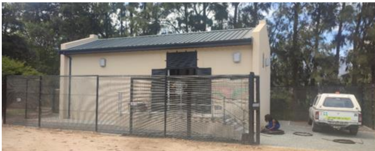
La Terra 11kv Switching Station
