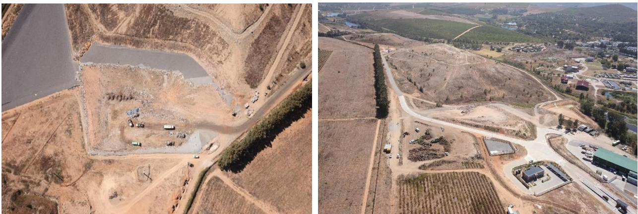
Landfill gas extraction
