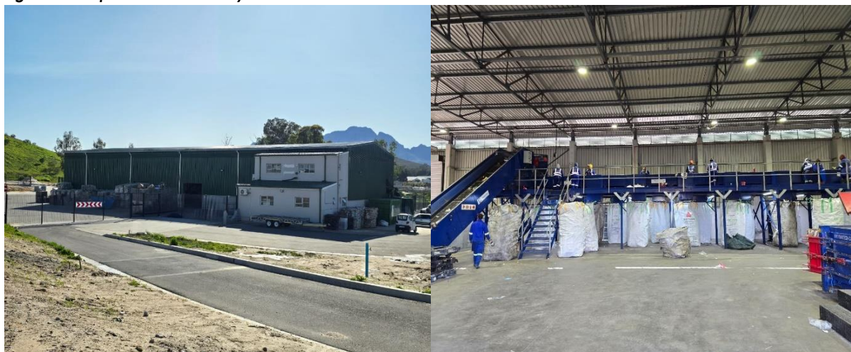
Figure 17: Operations underway inside the MRF
