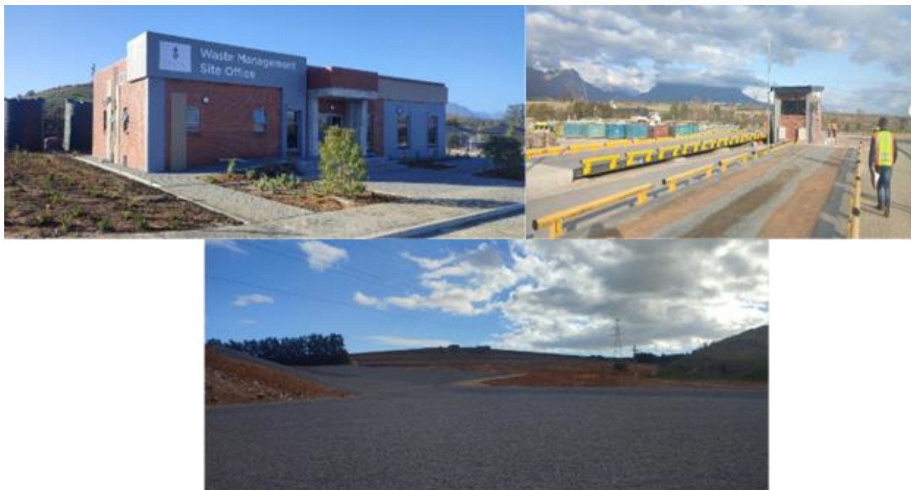
Stellenbosch Landfill New Cells and Associated Infrastructure
