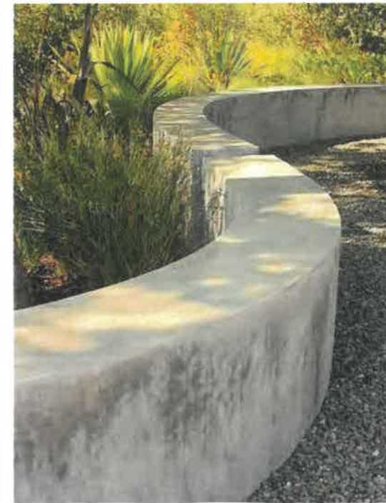
Low concrete walls
