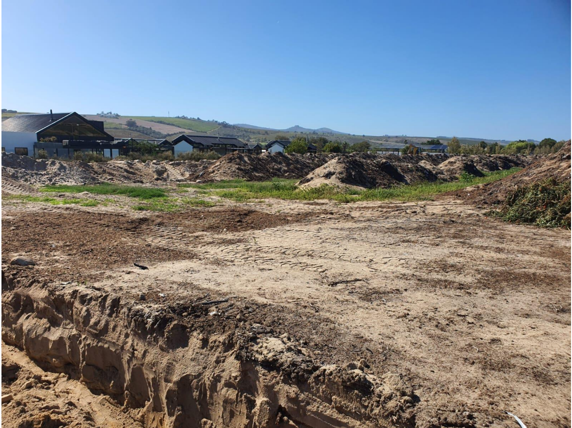
Photo 2: Additional windrows that were noted during the follow-up inspection.
