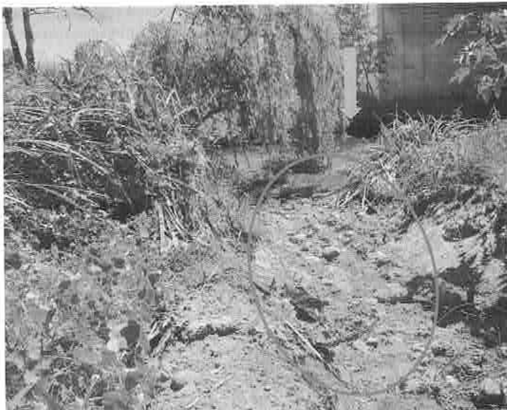
Photo 8: depicts excavation/earthmoving activities (area circled in red) that has been undertaken within the river (indicated by the yellow arrow).
