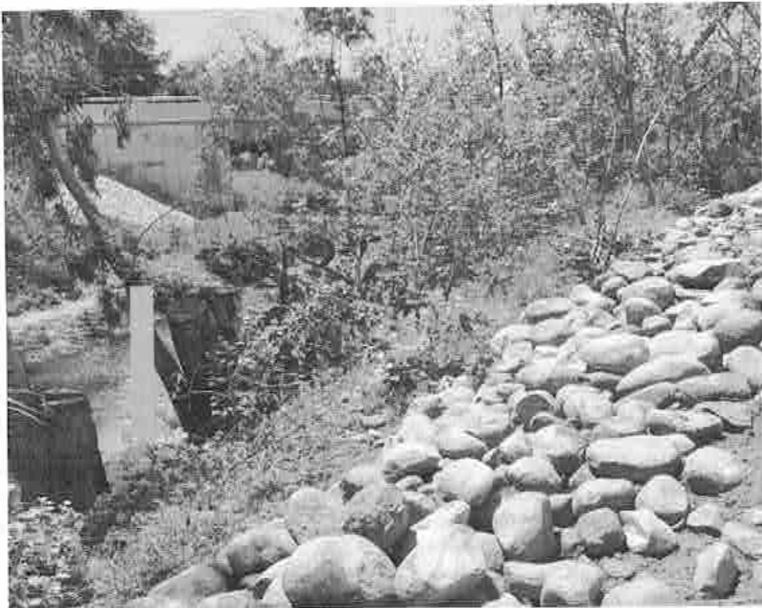
Photo 3: placement of rocks within the riverbank (indicated by the yellow arrow).
