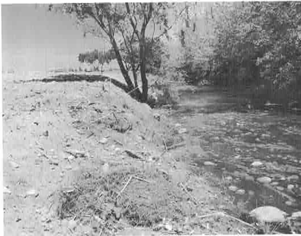
Photo 5: depicts earth moving/infilling activities that has been undertaken within the river.
