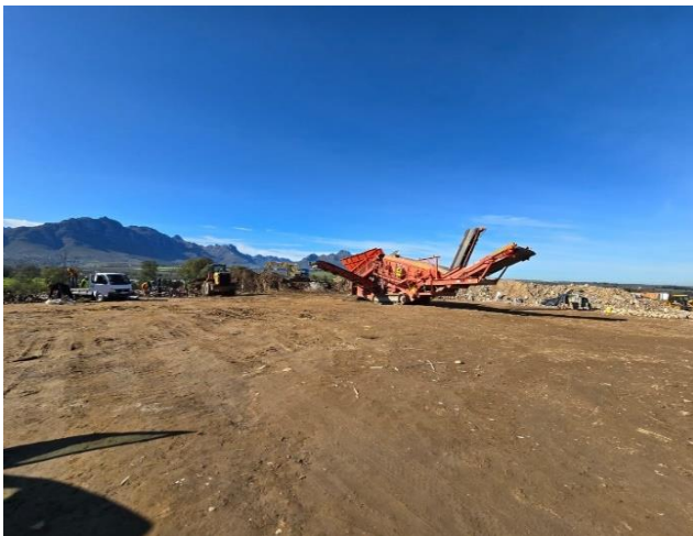
Crushing of builder's rubble
