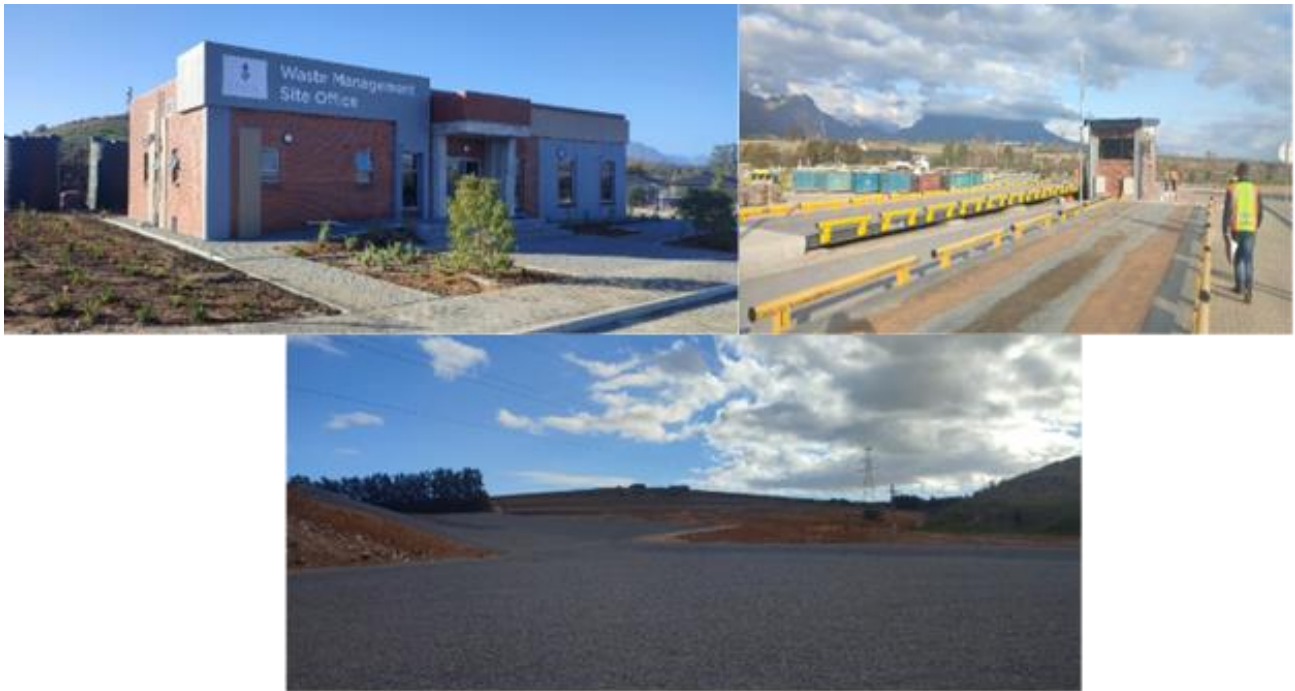
Stellenbosch Landfill New Cells and Associated Infrastructure
