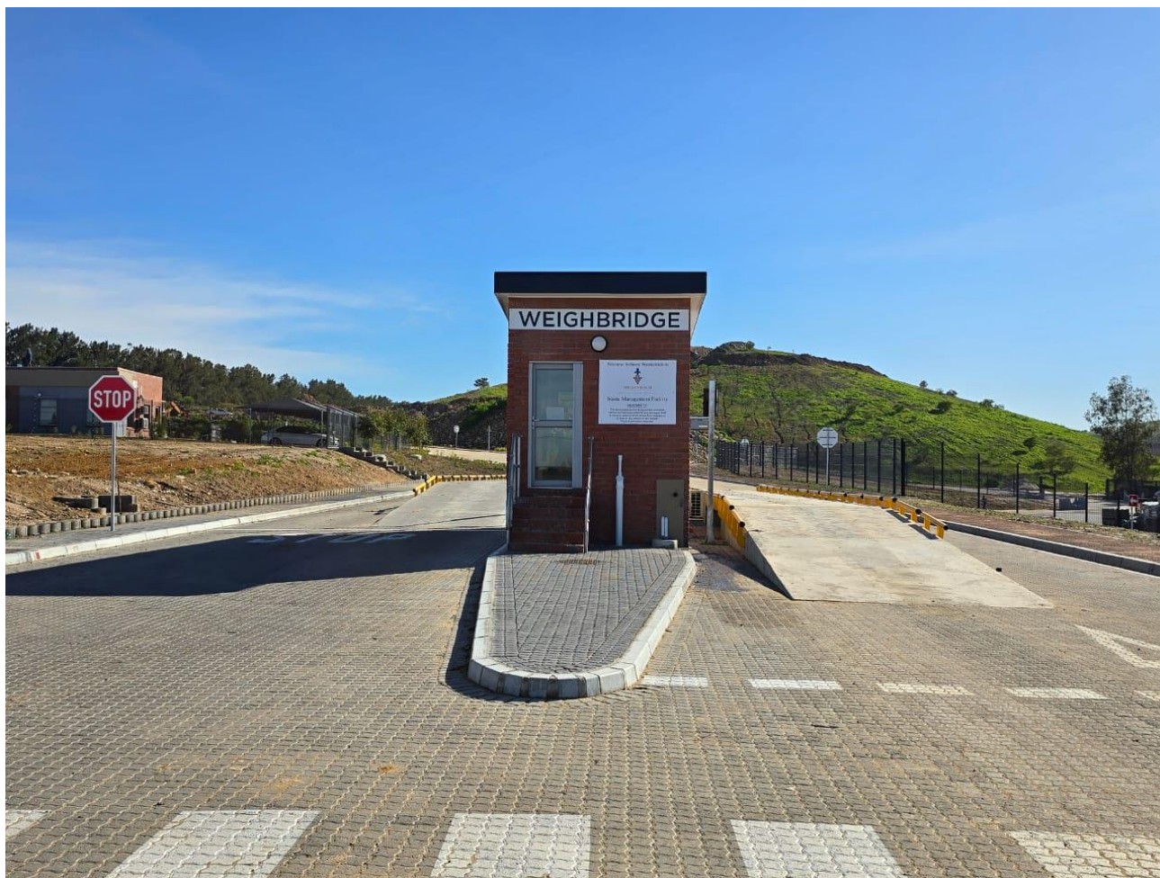
Weigh Bridge at the Landfill Site
