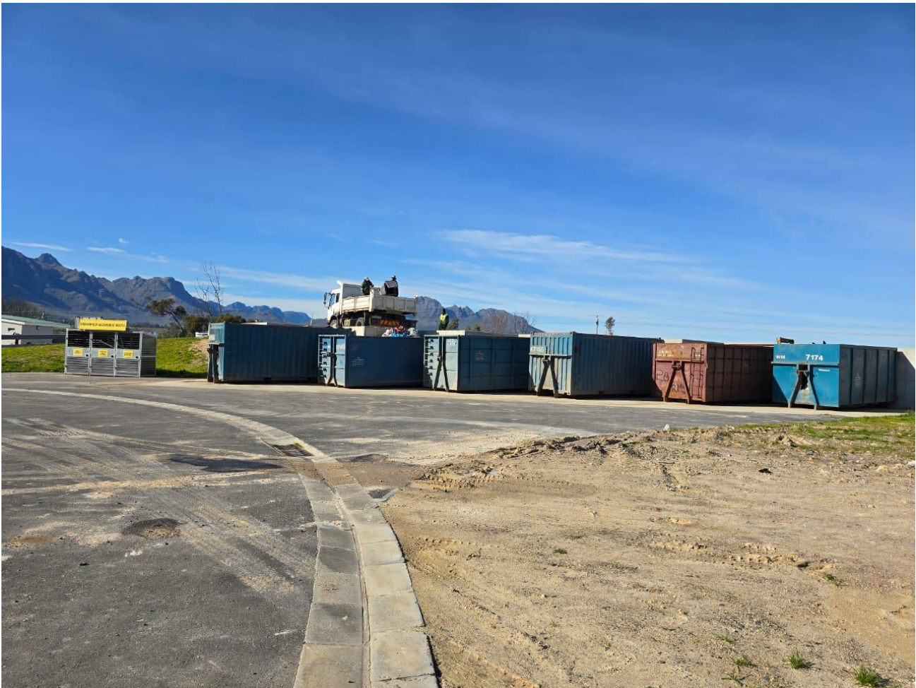
Public Drop-off Area
