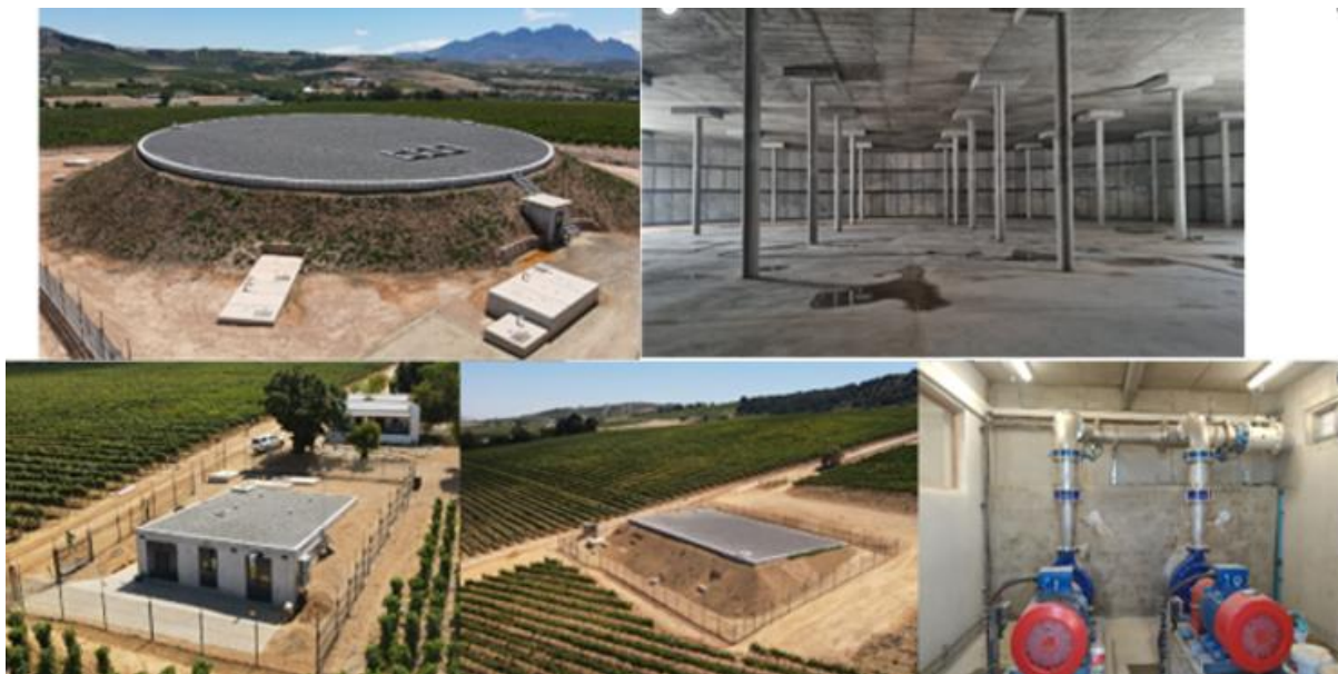
Construction of a new Reservoir and Pipeline: Vlottenburg – Phase 1 water will be provided to Polkedraai, Digtebij, Longlands and surrounding farms.
