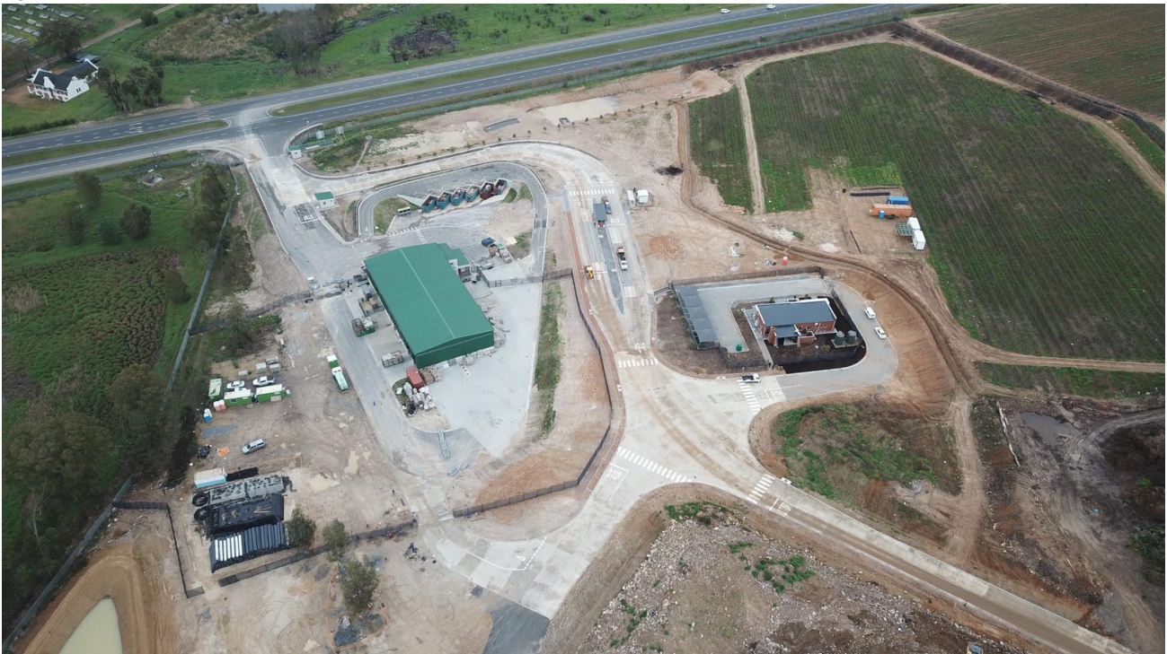
Figure 14: Material Recovery Facility (MRF)
