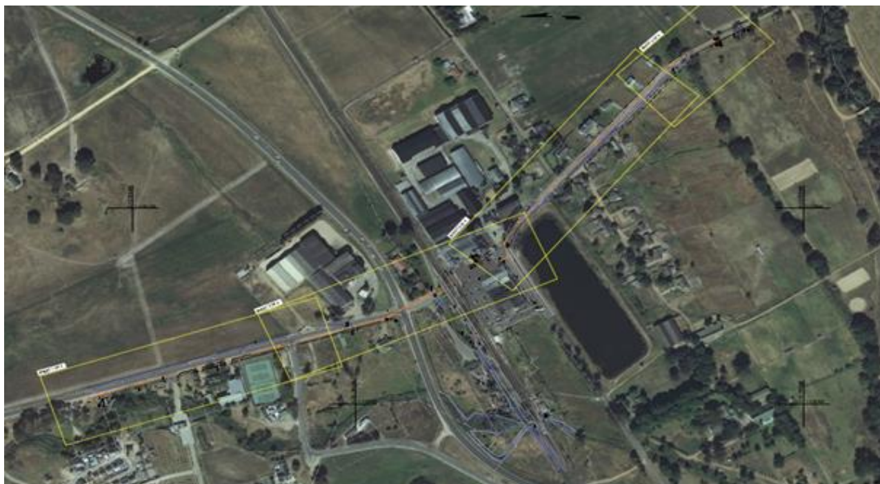
Vloffenburg Outfall Sewer Project Overview Image
