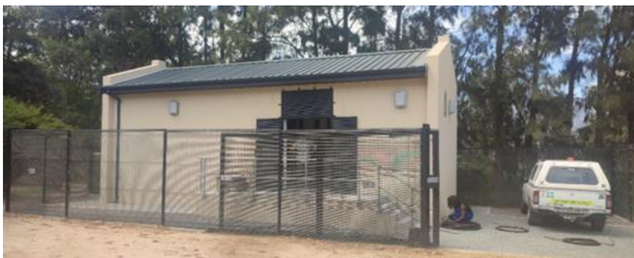
La Terra 11kv Switching Station
