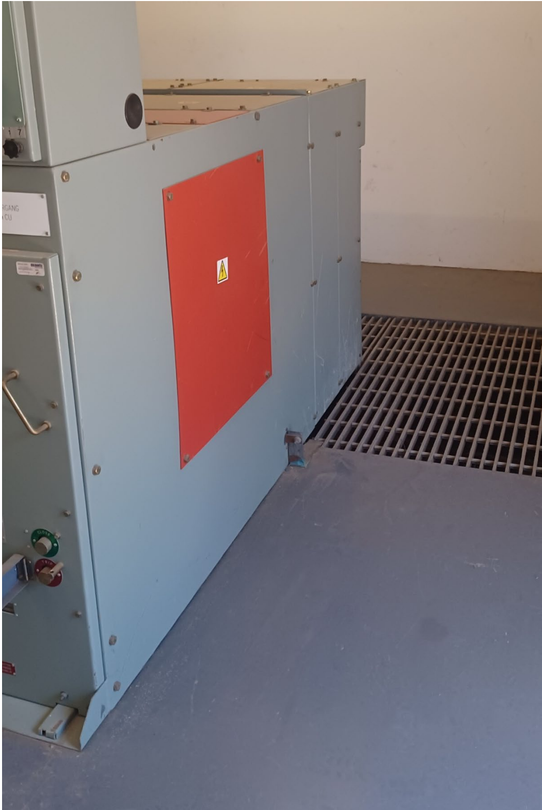
Figure 9-3: Space for 1 Additional Actom SBV 4 Panel
