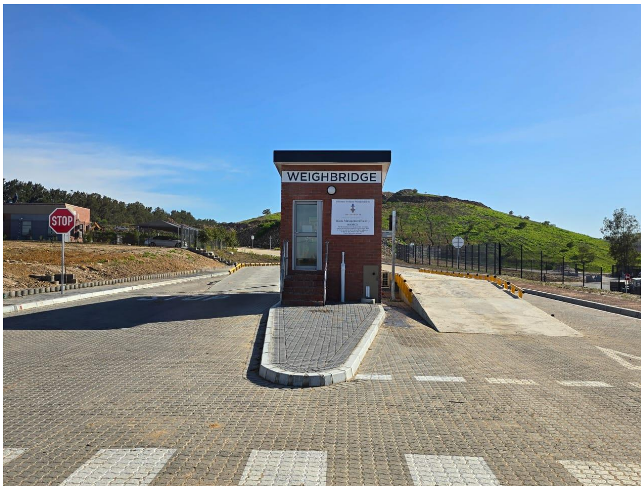
Weigh Bridge at the Landfill Site
