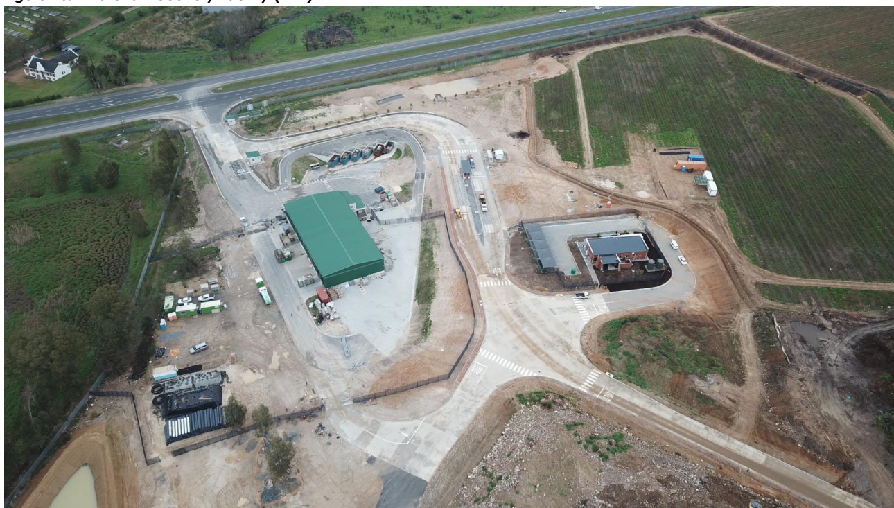
Figure 16: Material Recovery Facility (MRF)
